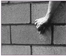
masonry for an extended time as they will become difficult to remove. Non-metallic scrapers may be required to avoid damaging the surface of clay masonry units or architectural block units. Often a small piece of a similar unit will function as a satisfactory scraper. (IMG13635) • Cover the Top:
