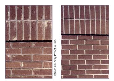
Careful selection of cleaning agents and techniques is required to remove mortar smears like these (left) without damaging units or mortar (right). (IMG13637, IMG13638)
