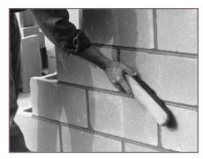
Clean As-You-Go: Remove mortar protrusions or droppings from masonry surface after mortar has set to avoid smearing mortar into masonry, but do not leave mortar droppings on
