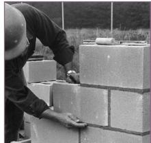
• Trim with Trowel: After tooling, use trowel to trim mortar burrs off flush with the face of the wall. (IMG13633)
