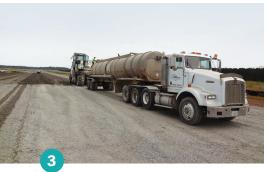
Mixing cement and water into pulverized runway
