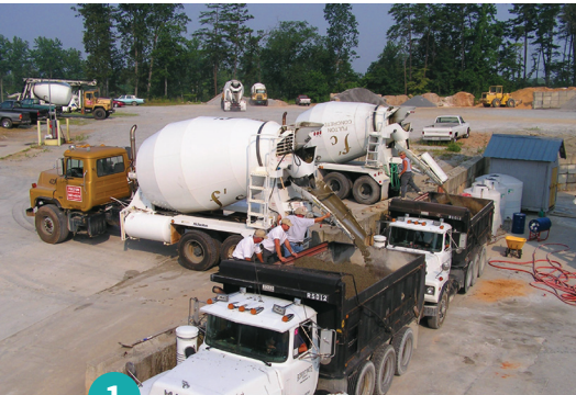
1 Ramp elevates ready mix truck higher than dump truck.
