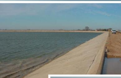
Soil-cement shown above at normal operating pool, following reservoir refilling.
