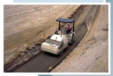
Vibratory compactor shown compacting soil-cement lift.
