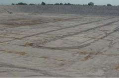
Soil-cement placement completed in one cell prior to refilling.
