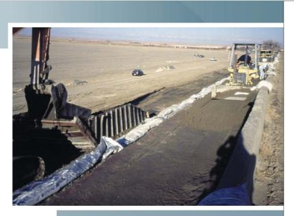
Soil-cement placement operations adjacent to existing concrete parapet at crest of dam.
