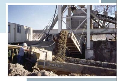
Soil-cement batch plant located within drained reservoir.
