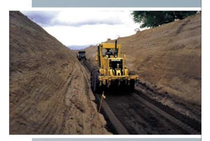
First lift of soil-cement being spread at elevation of maximum scour depth.
