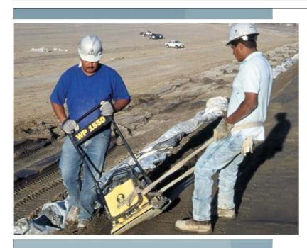
Compacting sloping soil-cement step face with vibratory plate compactor.
