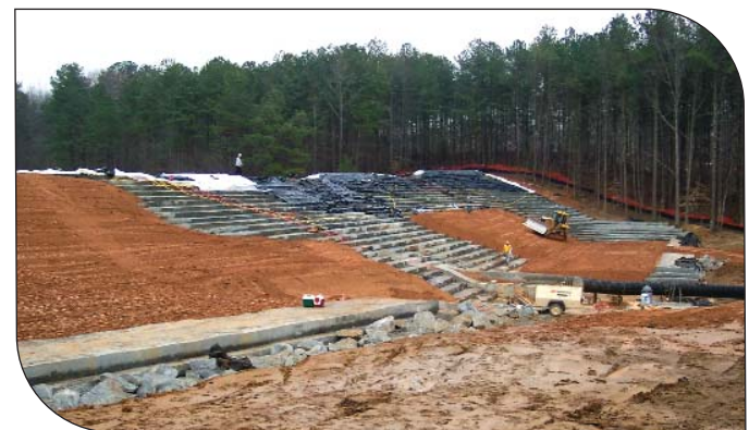
Placement of earthfill over the completed RCC spillway.
