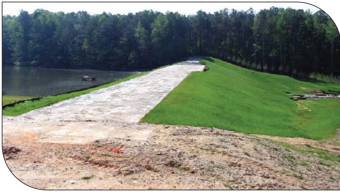
Completed project with grass covered downstream slope.
