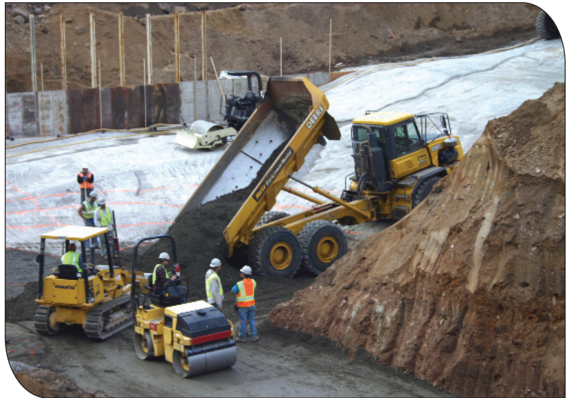
Equipment used to transport, spread and compact RCC
