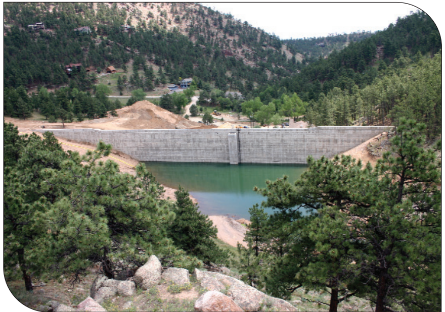
A view looking at the upstream face of the dam during initial filling
