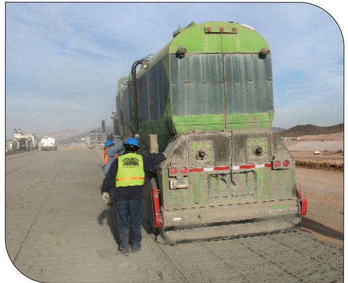
Spreading cement.
