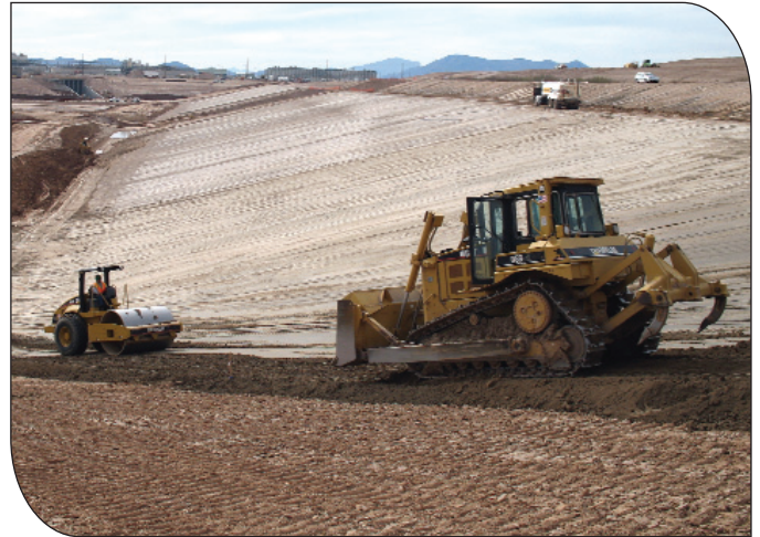
Spreading and compacting soil-cement.
