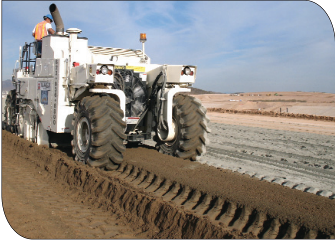
A pulverizer mixing soil-cement.
