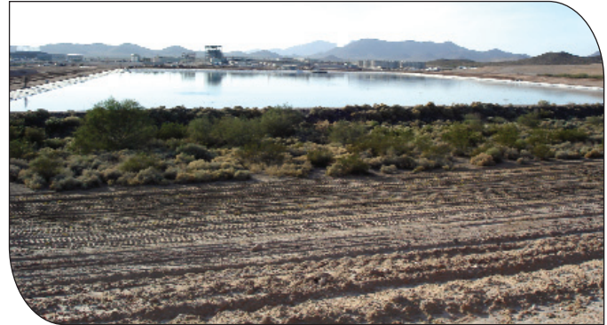
General view of reservoir in operation.
