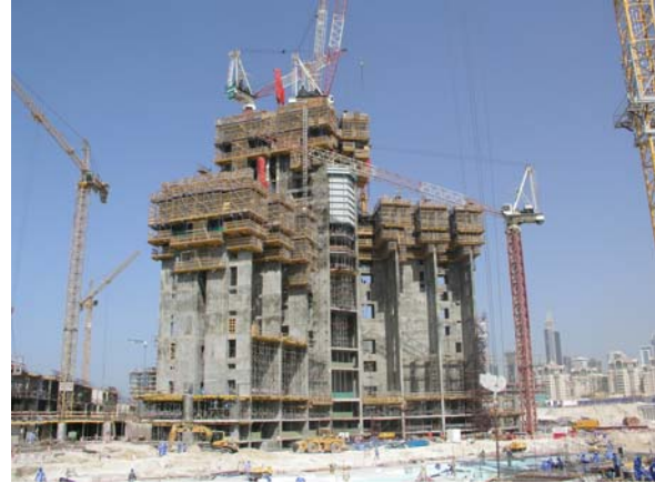
Figure 23 – Self-Climbing Formwork System
