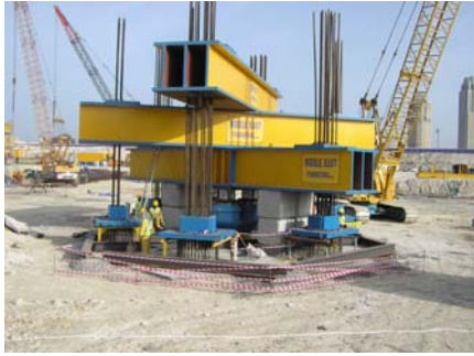
Figure 12 – Test Pile (6,000 tonnes)
