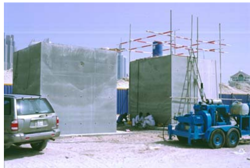
Figure 11 – Raft Conc. Placement Test Cubes
