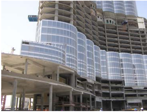
Figure 8 - Reinforced Concrete Structure
