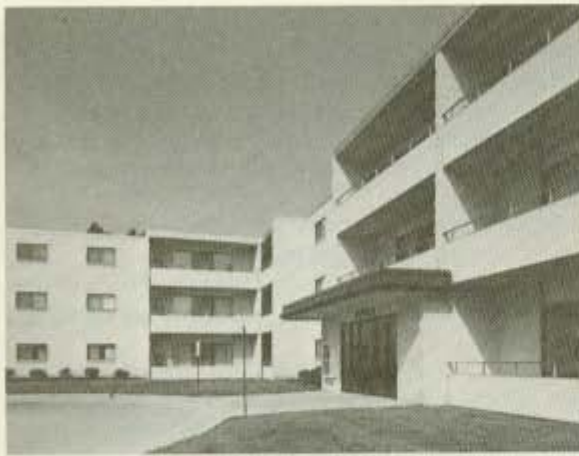
Many firesafety-conscious communities are insisting upon fire-resistant construction for low-rise apartment buildings. The concrete floors and masonry in this building resist fire, reduce property loss, and protect residents. (Photo: © Thom Abel 1978)
