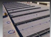
Figure 1 (above): Two 89 x 89 x 6-mm  $(3^{1/2} x 3^{1/2} x 1/4-in.)$ angle irons spaced about 1 m (3.5 ft) apart were embedded in each slab for electrodes in a backto-back fashion. (IMG14730)
