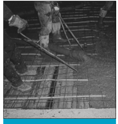
Fig. 3. Concrete is placed over tubing for a radiant floor.
