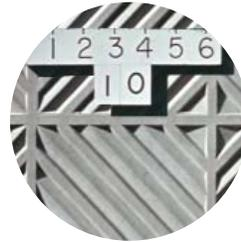
**Panel 10:** This panel is a forerunner of today's wide array of formliners. Sharp edges were softened over the years by minor paste erosion. (IMG14238)
