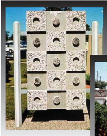
**Panel 4:** Polystyrene blockouts and chemical retarders allowed for surface textures, and lightweight concrete was used for the back-up. Many formed surfaces are still done in much the same way. (IMG14225)
