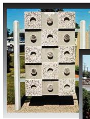
Panel 4: Polystyrene blockouts and chemical retarders allowed for surface textures, and lightweight concrete was used for the backup. Many formlined surfaces are still done in much the same way. (IMG14225)
