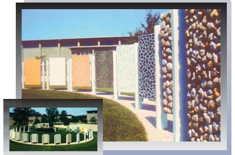
Figures. In 1962, newly erected panels at PCA's property near Chicago put bright new faces on concrete surfaces. The display consisted of a circular walkway in exposed aggregate concrete, and white cement concrete posts supporting two panels placed back-to-back. [IMG14306, IMG15614]
