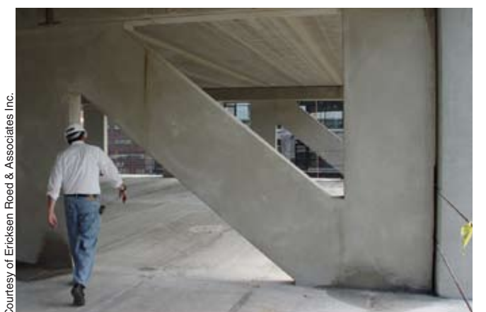
Fig. 10. Flag Builders' construction superintendent, Tom Casey, walks through a vertical element of new prestressed truss system. Vertical components of the truss system are eventually incorporated into the interior walls of the condominium units.
