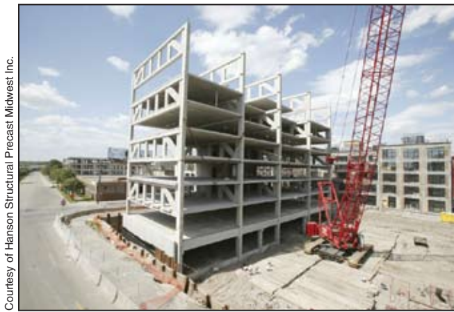
Fig. 5. The column-free space on the first-floor retail level of the Bookmen Stacks condominiums ensures that the owner has maximum flexibility and space for layout of shops and large open areas, a critical advantage in the real estate market.
