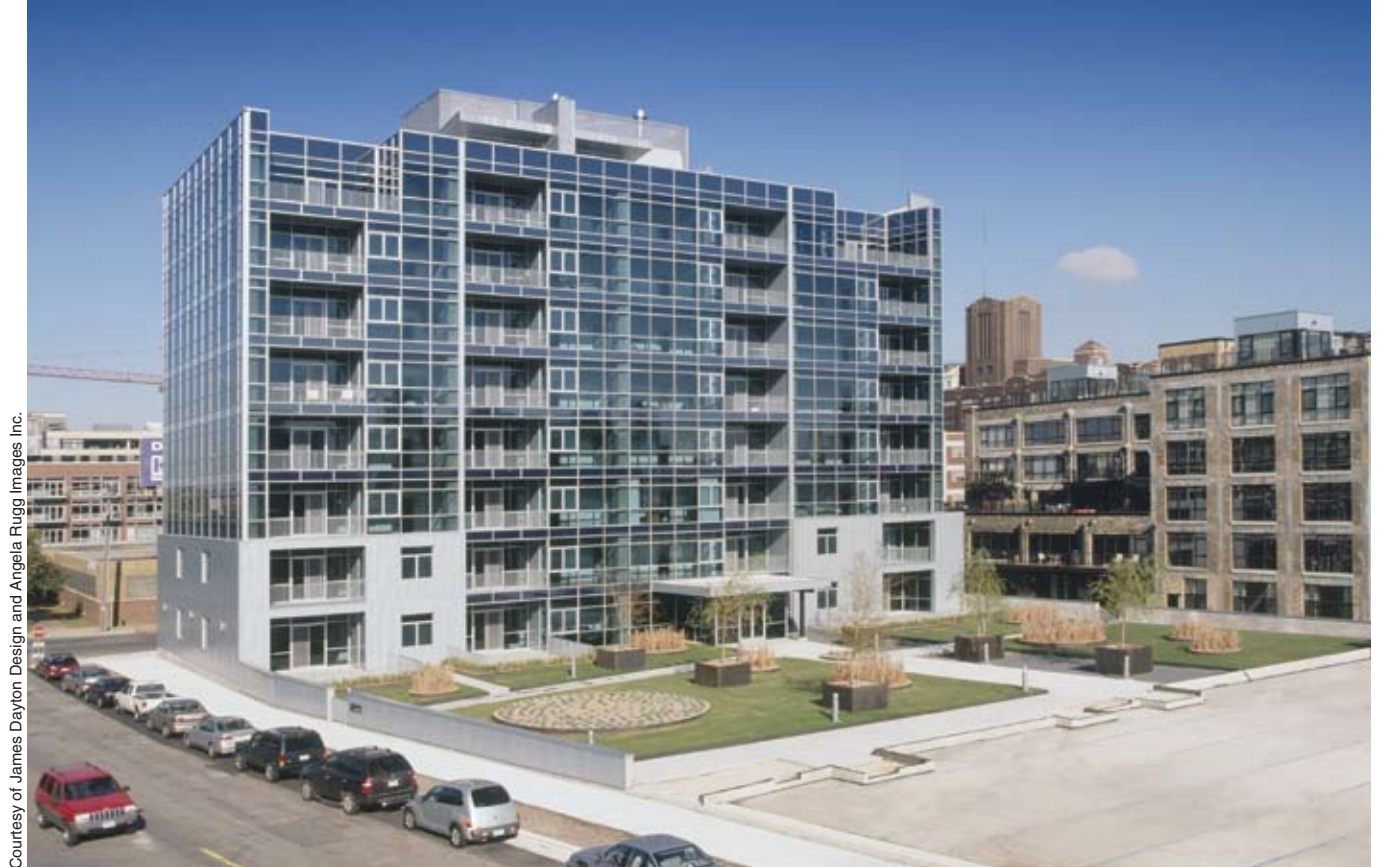
Fig. 18. The Bookmen Stacks condominium's (Lofts at far right) landscaped courtyard serves as a gathering space for the entire Bookmen campus. The concrete structure is visible from the outside through a transparent glazing system that wraps the exterior.
