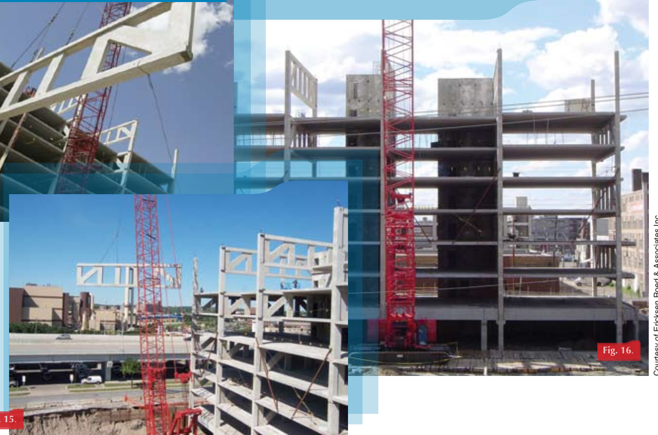
Fig. 16. This photo perspective is an overall view of the ER-POST system. All but the two final trusses are in place, and precast concrete plank (12 in. [300-mm] thick) will soon establish the top two floors. The parking is clear-spanned with precast, prestressed concrete double tees. The truss bottom chord supports the second floor, and the truss top chord supports the third floor, leaving the first floor completely open. The erection is fast and simple, and with all precast concrete elements—columns, trusses, and plank—the onsite work is minimized. With this building elevation, one can visualize the amount of open space on all floors, allowing for large flexible space planning.
