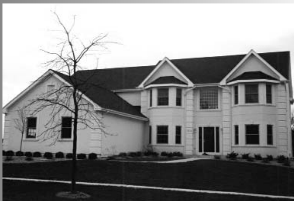
(Top) Tom Hanley of Energy Block Inc. built this ICF home in Mundelein, Illinois.
