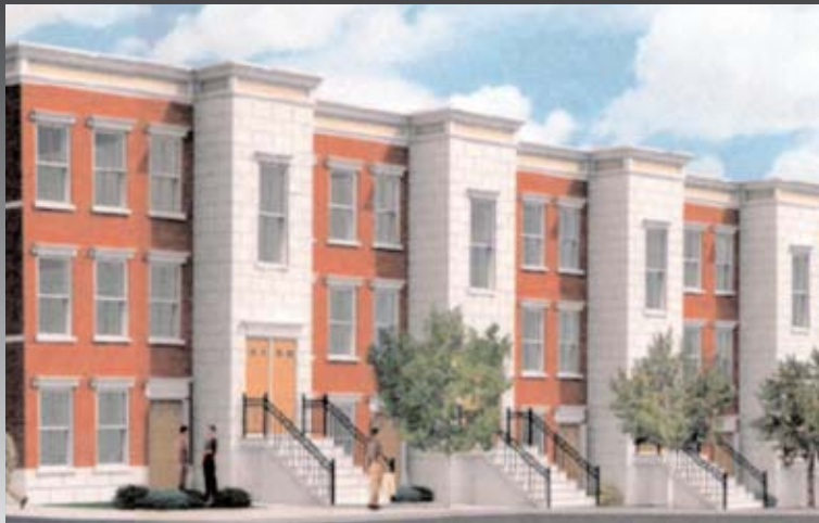
Melrose Commons II features precast concrete structures that provide the energy savings of an Energy Star home.
