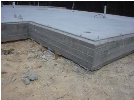
SLABTEK foundation after lift
