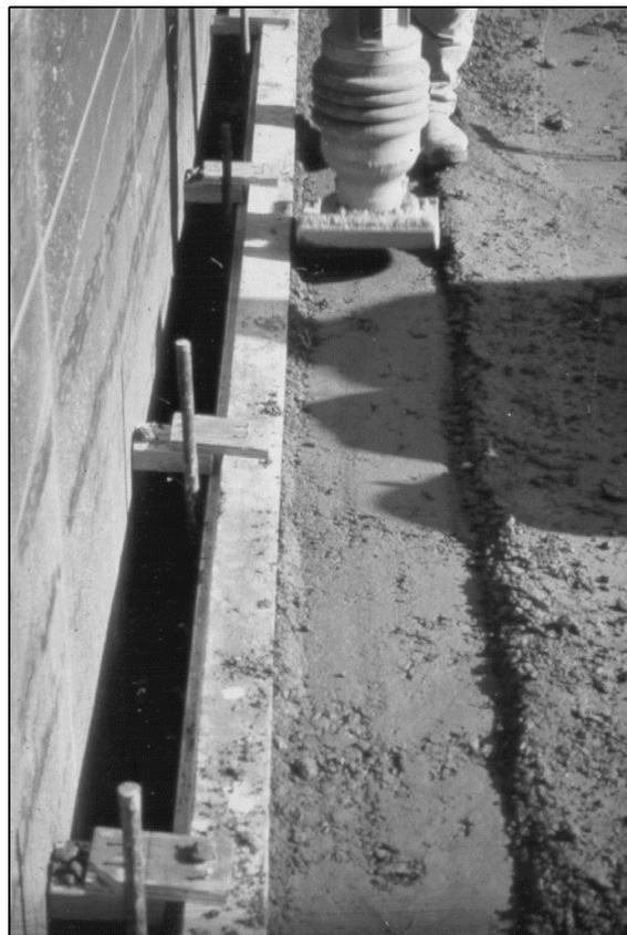
**Figure 5.2**—RCC compaction in confined area using a “jumping jack” type compactor.
