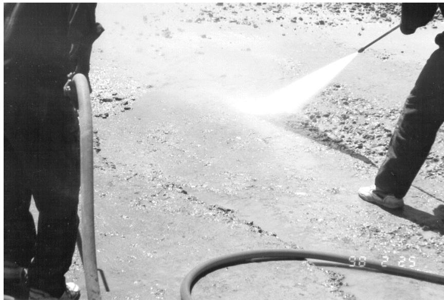
**Figure 5.5**—RCC surface preparation using high-pressure air-water.
