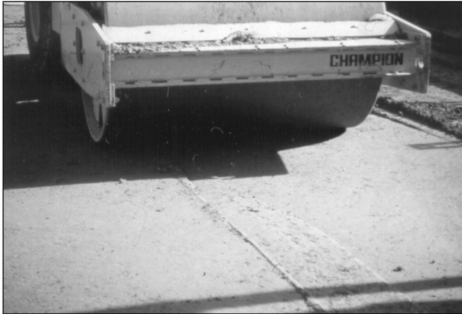
**Figure 5.1**—RCC surface during compaction with a smooth-drum vibratory roller.
