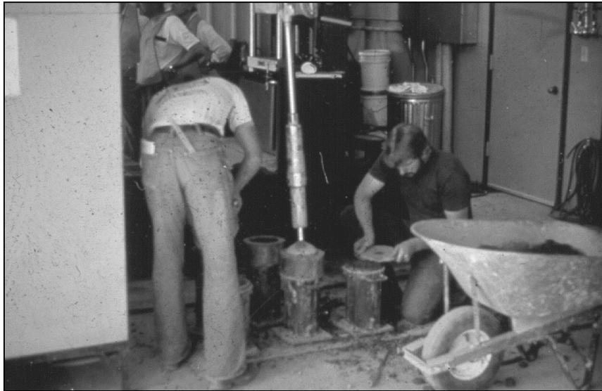
**Figure 4.2**—Preparation of RCC cylinders with a vibrating hammer
