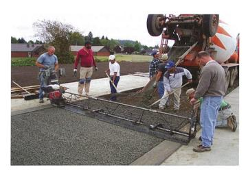
Figure 11. Pervious concrete is usually placed and then struck off with a vibratory screed. (R. Banka)
