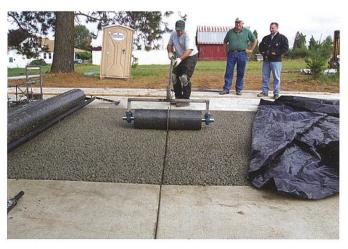
Figure 14. Joint roller, commonly referred to as a "pizza cutter." (R. Banka)
