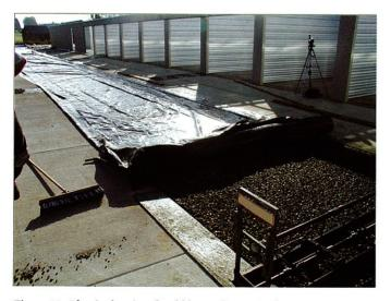
Figure 15. Plastic sheeting should be used to cover the pervious concrete and be installed within a few minutes of consolidation to prevent moisture loss. (R. Banka)
