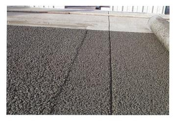
Figure 12. Pervious concrete after screeding (left) and after compaction (right). Note the joint aligned with previously placed slab to avoid reflective cracking. Roller used for compaction is visible on the far right. (R. Banka)
