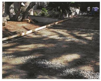
Figure 8. Preparation for a sloped installation. Crushed rock drains at intervals down the slope direct water away from the pavement and prevent water from flowing out of the pervious concrete (See also Figures 9 and 10). (S. Gallego)
