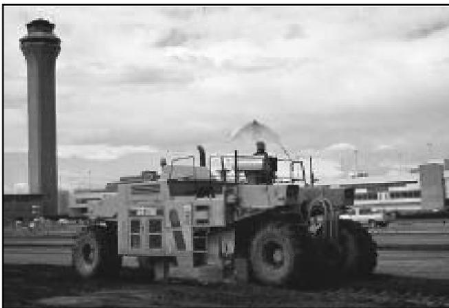
***In-place mixing for cement-modification of clay subgrade at Denver International Airport.***
