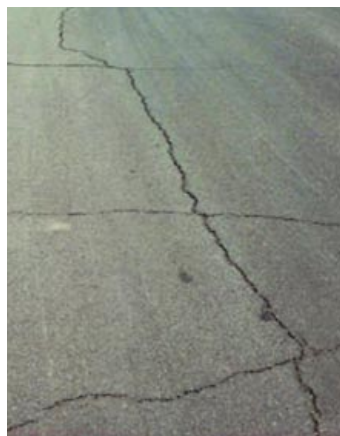
Reflection Cracking
