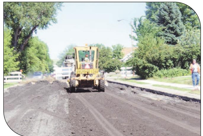
**A grader was used to place the new cement-stabilized base, consisting of the pulverized asphalt and old base material.**
