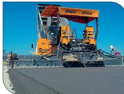
Asphalt type paving equipment is used to place RCC pavement at the Hyundai auto manufacturing facility in Montgomery, Ala.
