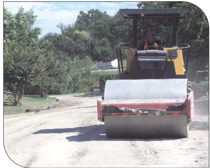
Steel-wheeled vibratory roller compacts the reclaimed base to 95% standard Proctor density.
