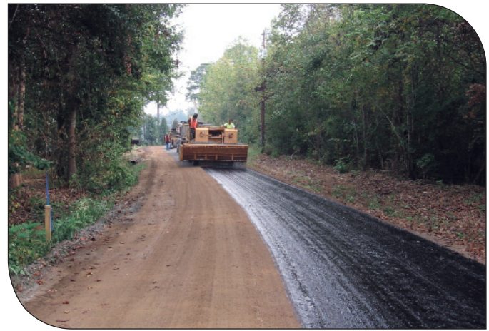
Application of bituminous surface treatment (chip seal).
