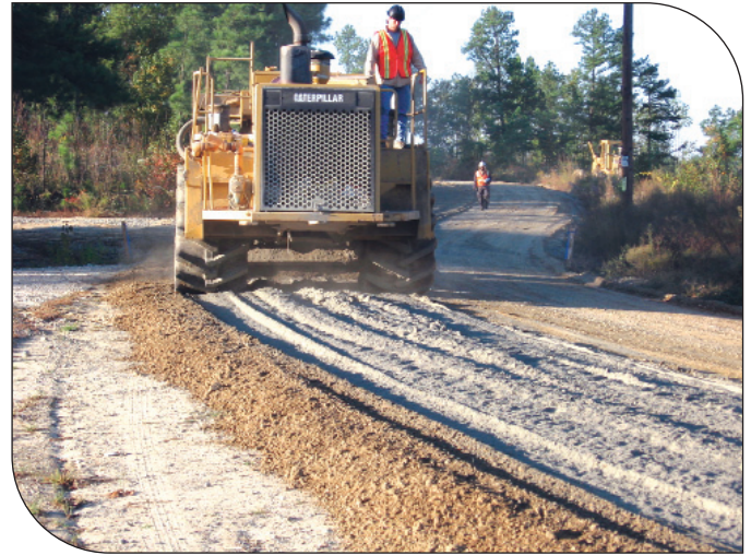
Mixing cement during the FDR process.
