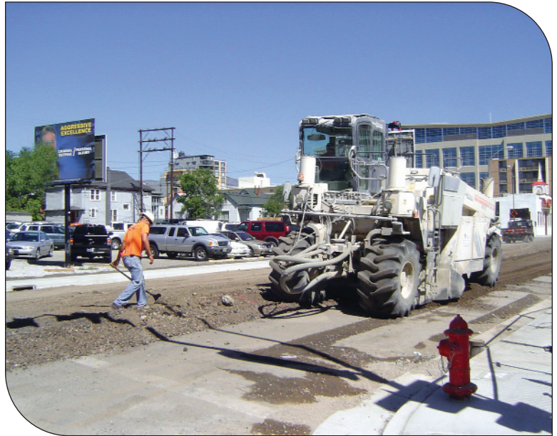
Pulverizing failed flexible pavement in downtown Reno, Nevada.
