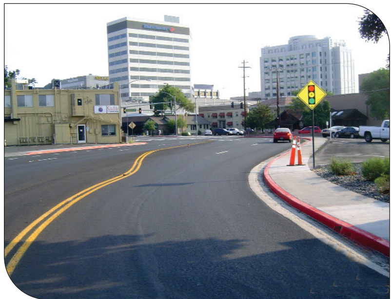
Sierra Street after reconstruction using FDR with cement.
