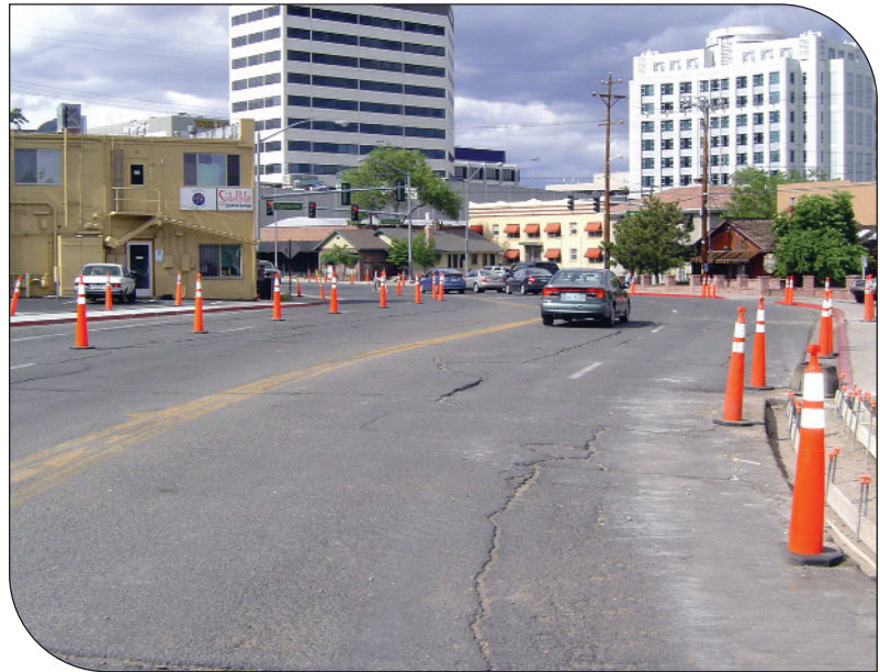
Sierra Street prior to reconstruction.
