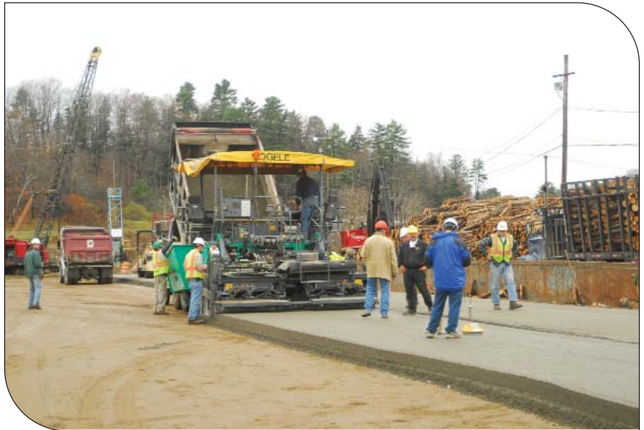
Vögele high-density paver and density testing with nuclear gauge.
