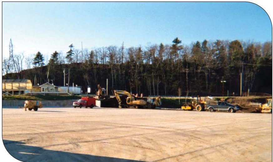
RCC pavement after construction.
