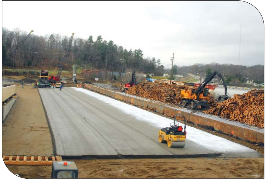
Rolling and curing operations during construction.
