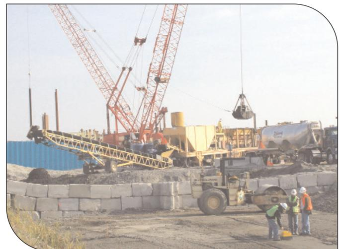
Dredged sediment placed directly into pugmill mixer. Foreground: Treated sediment compacted to form new land.
