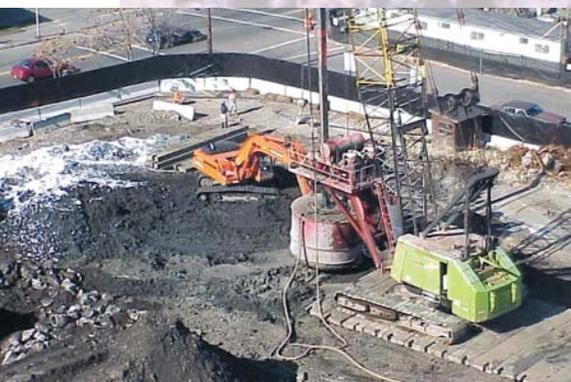
*MGP byproducts including DNAPLs and LNAPLs treated in-situ with cement-based S/S.*
