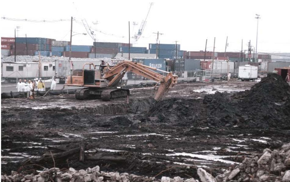
Best Demonstrated Available Technology (BDAT) for over 50 RCRA-listed hazardous wastes. The technology has found increasing use at brownfield remediation projects due to the ability to reuse S/S-treated soil as an engineered fill or pavement base.
