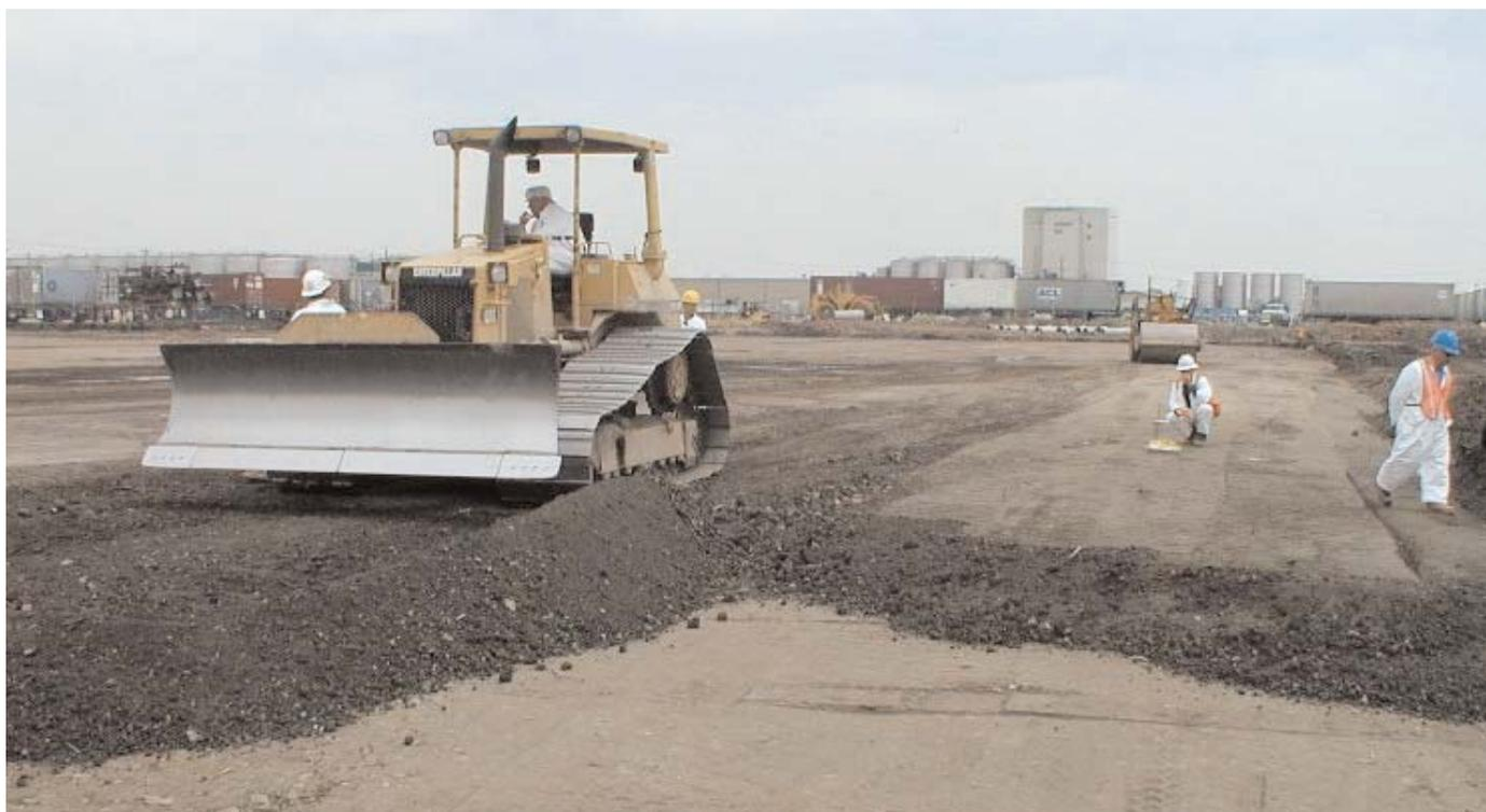
Approximately 23,000 cubic meters (27,000 cubic yards) of arsenic-impacted surface soil were stripped from the surface of the site up to a depth of 0.6 meters (2 feet). This soil was mixed with cement and mixing water in a mobile pugmill erected at the site. A conveyor scale on the pugmill equipment ensured that 8% (by weight) cement was mixed into the soil. A total of 3,900 metric tons (4,300 short tons) of cement were used in this process.
