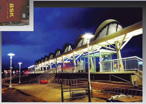
Figure 1 (above). Shawnessy Light Rail Transit Station, Calgary, Canada.
