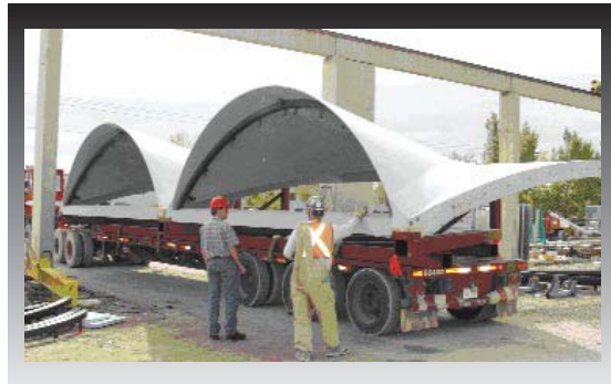
Figure 3. Canopies ready for transportation.
