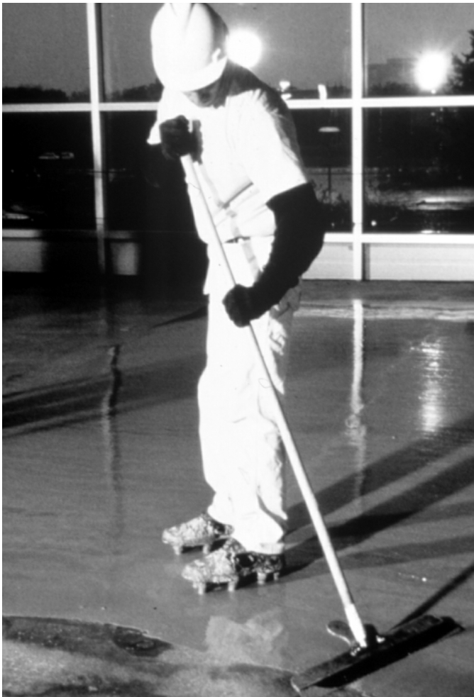
Figure 13. Self-leveling toppings can be used to restore the floor surface on an otherwise sound slab. Underlayments usually require a floor covering material such as tile or carpet. (69682)
