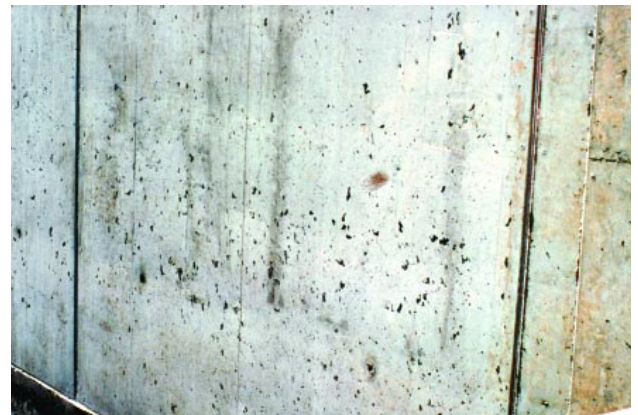
Fig. 24. Surface air voids, or bugholes, are small cavities of entrapped air bubbles in the surface of formed concrete. (70154)
