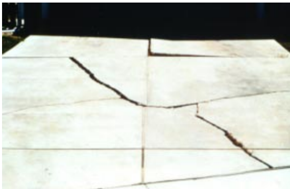
Fig. 23. Settlement can cause a variety of problems in concrete structures, from cracking and performance problems to structural failure. (56521)
