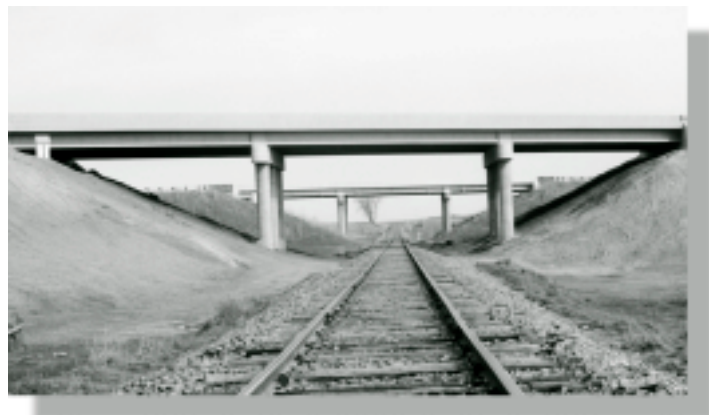
High strength concrete allowed the number of girder lines to be reduced from five to four.
