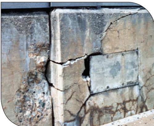
**Figure 3. This parapet wall has been severely affected by ASR. Notice the cracking, joint closing, spalling of concrete surfaces, and lateral offset that have developed. (IMG12295)**
