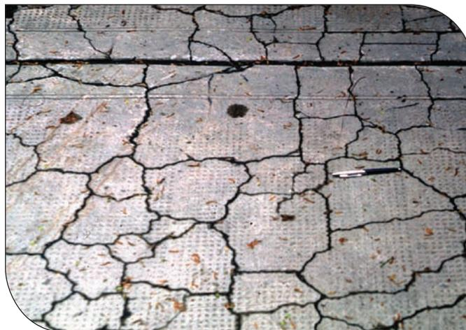
**Figure 21. Map cracking pattern caused by ACR (IMG12982).**
