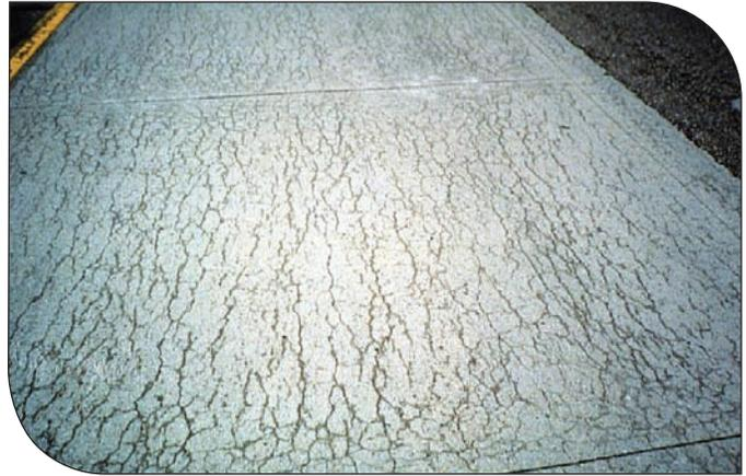
**Figure 4. Longitudinal cracks induced by ASR in a concrete pavement. (IMG21371)**
