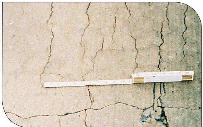
**Figure 5. Close-up view of well developed cracking in a pavement, a typical pattern associated with ASR. The prominent cracks are in a longitudinal direction as there is less restraint to lateral expansion. (IMG13049)**
