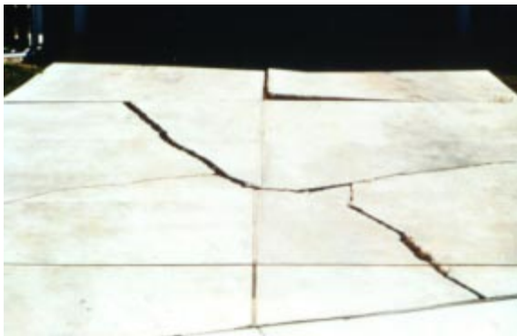
Fig. 23. Settlement can cause a variety of problems in concrete structures, from cracking and performance problems to structural failure. (56521)
