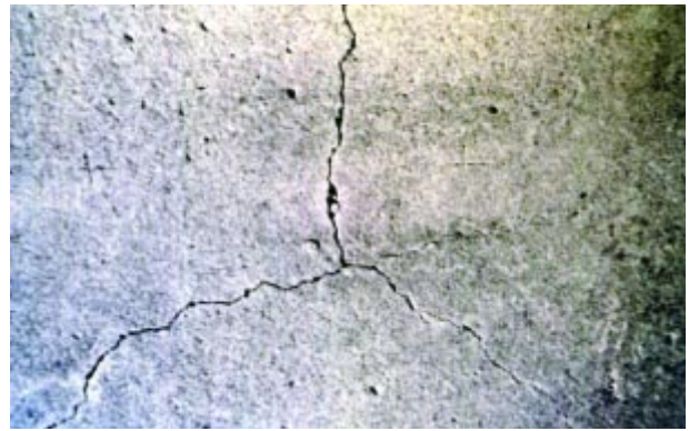
Fig 21. Restraint to drying shrinkage is the most common cause of concrete cracking. (A5271)
