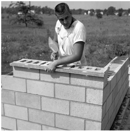
Fig. 5. (a) The mason checks corners for alignment,
