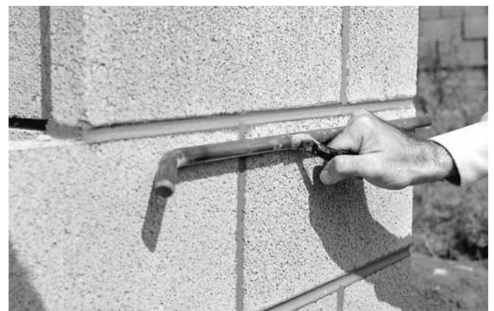
Fig. 11. Proper tooling yields a dense, weather-resistant mortar joint surface and a neat, uniform appearance.
