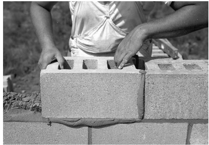
Fig. 3. A well-filled head joint results from mortaring both block.
