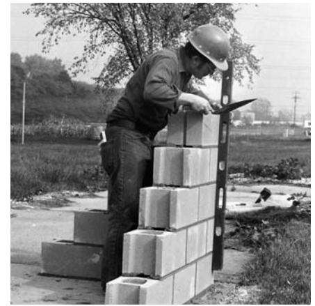
(c) and for being plumb.
