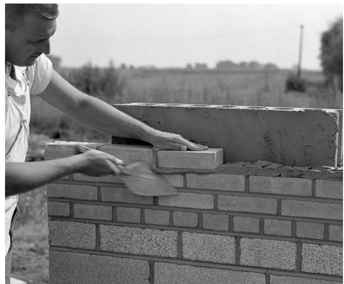
Fig. 4. Mortar extrudes from the joints of a unit being placed, indicating full mortar joints.
