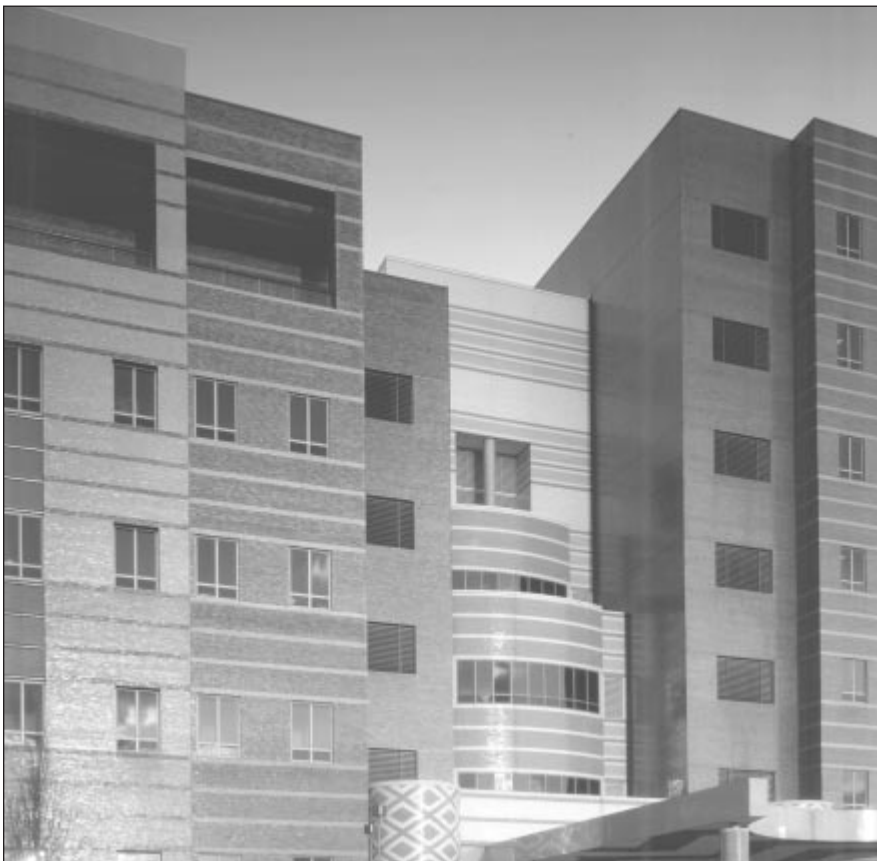
Architects Smith, Hinchman & Grylls used mortar cement mortar and brick of differing color and texture to define distinct building areas within a unified visual theme on the Veterans Administration Hospital in Detroit.
