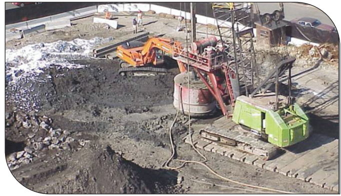
Soil mixing with auger
