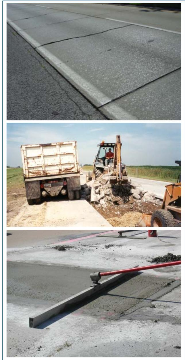
Figure 10-1. Full-depth repair of a concrete pavement slab
