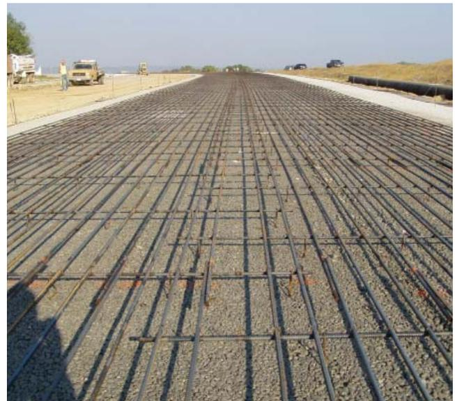
Figure 1-8. CRCP reinforcement placed before paving
