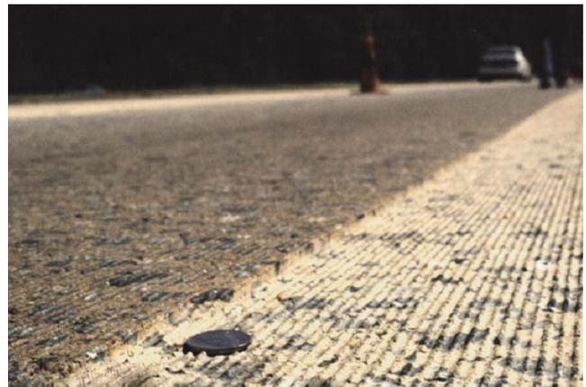
Figure 10-7 Diamond grinding concrete pavement for surface restoration
