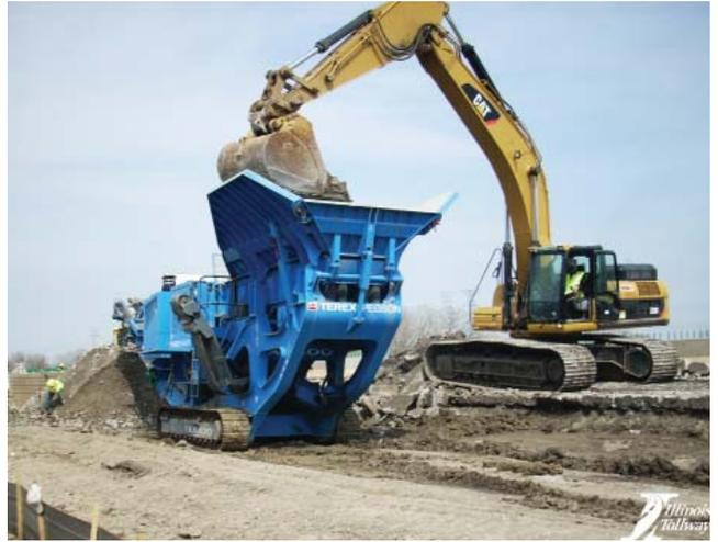
Figure 9-4. Existing concrete recycled in-place and reused for base material on the Tri-State Tollway in Illinois
