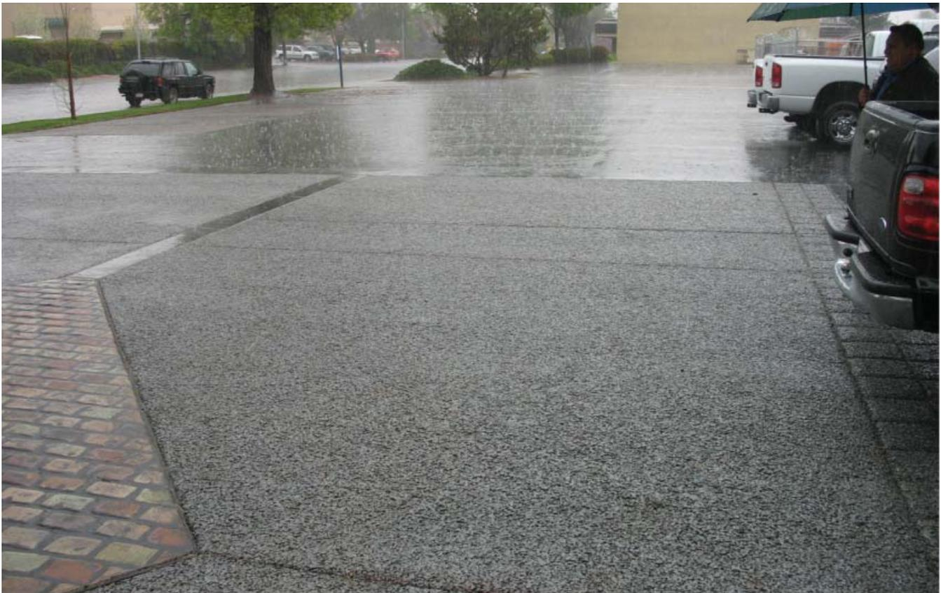
Figure 3-7. Pervious concrete pavement in the rain
