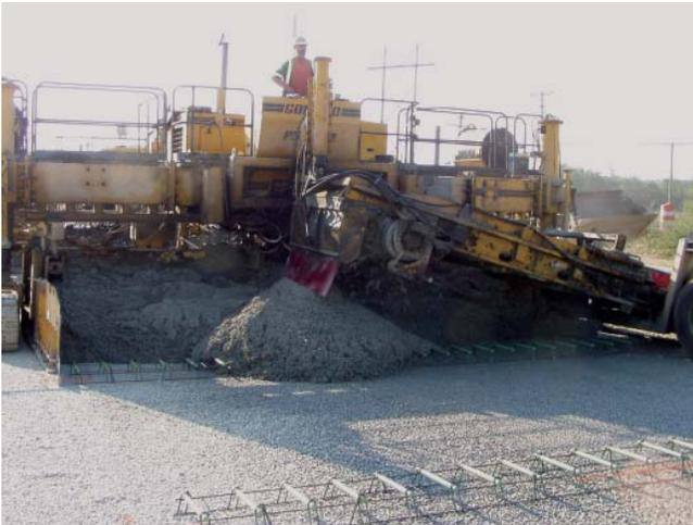
Figure 1-5. Concrete placed over dowel baskets
