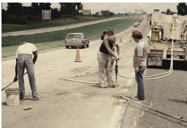
**Figure 10-4.** Drilling operation as part of slab stabilization
