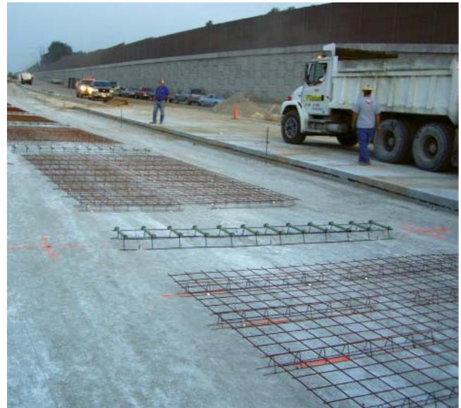
Figure 1-7. JRCP reinforcement in place before paving
