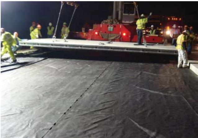
Figure 4-2. Nighttime placement of precast panels in Virginia
