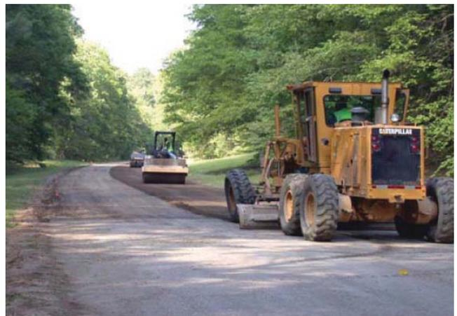
Figure 7-6. Equipment for compaction and finishing
