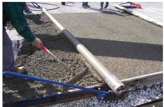
Figure 3-11. Compacting the placed pervious concrete
