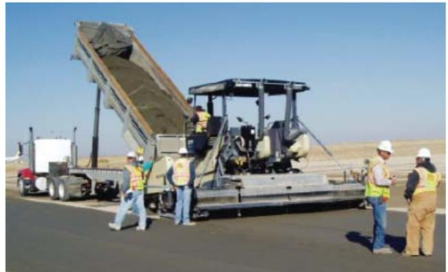
Figure 5-13. RCC placement
