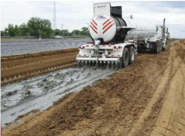
**Figure 8-2.** Cement slurry added to subgrade material (cement slurry is applied the same way for CTB and FDR applications)
