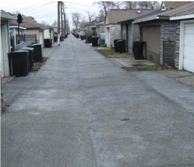
Figure 3-3. Pervious concrete for alley in Chicago, Illinois
