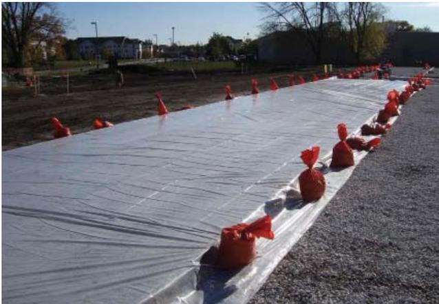
**Figure 3-12.** Curing pervious concrete with plastic sheeting
