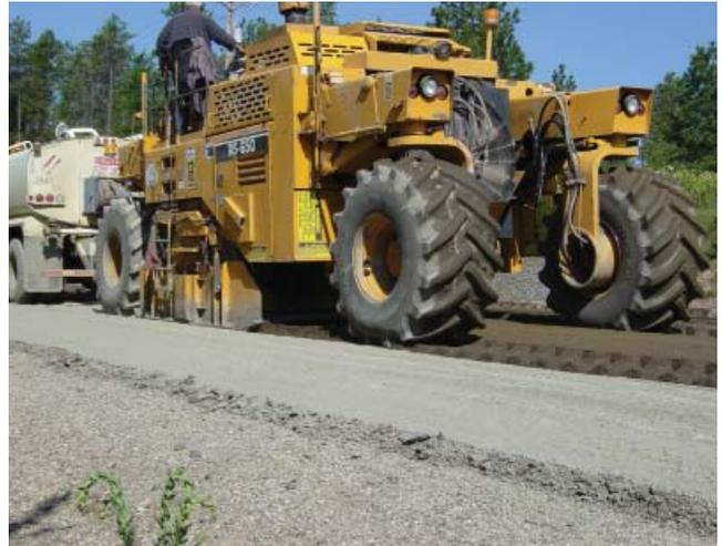
Figure 7-5. Mixing the cement into the pulverized material
