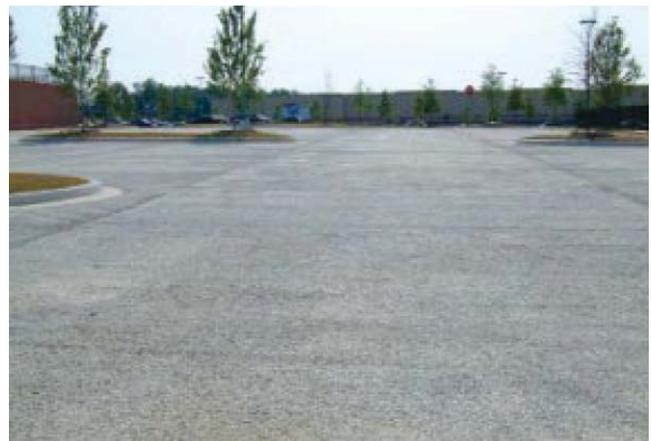
Figure 3-5. Pervious concrete pavement parking lot
