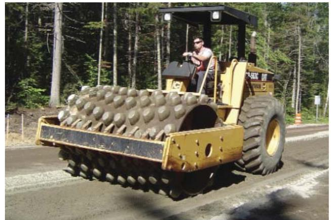
**Figure 8-4.** Sheepsfoot roller used for compaction
