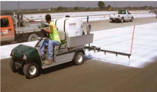
Figure 5-16. Curing RCC
