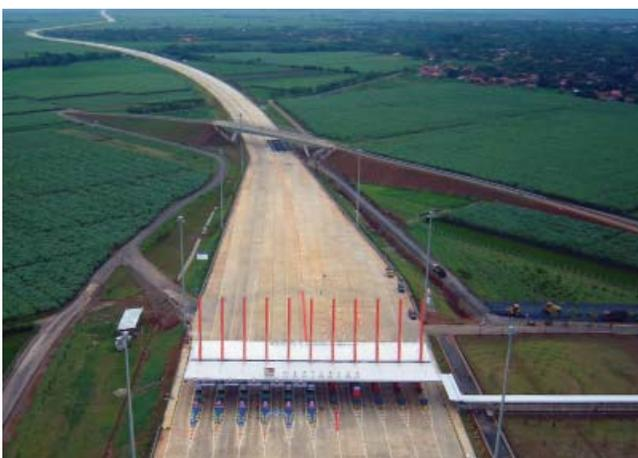
Figure 4-3. Precast pavement system in Indonesia
