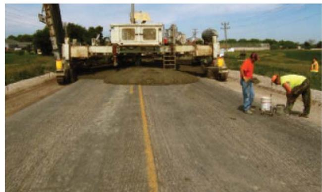
**Figure 2-5. Bonded overlay construction**
