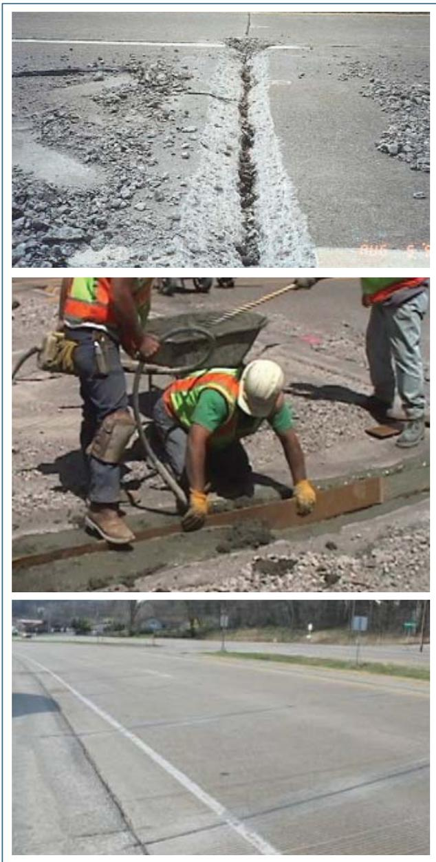
Figure 10-2. Partial-depth repair process at joint
