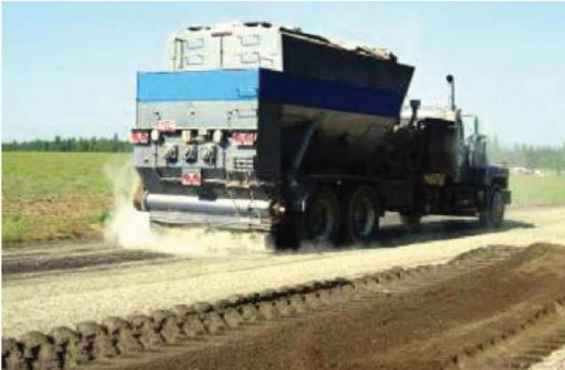
Figure 7-3. Dry cement placed on pulverized material
