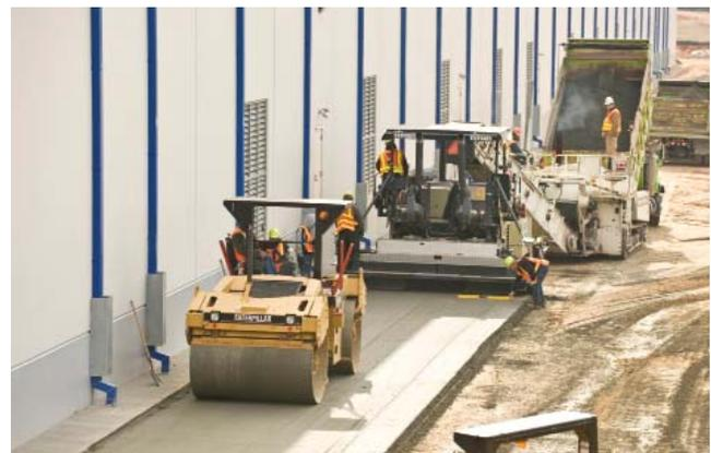
Figure 5-4. RCC construction for commercial and heavy industrial applications
