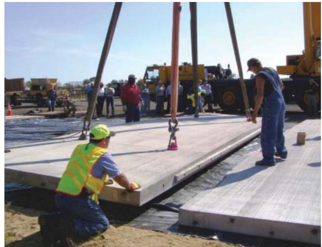
Figure 4-7. Placement of a prestressed precast panel
