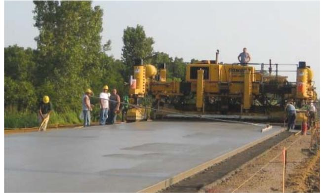
**Figure 2-6. Unbonded concrete overlay construction over a nonwoven geotextile interlayer**
