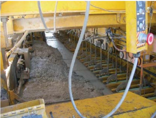
Figure 1-6. Dowel-bar inserter
