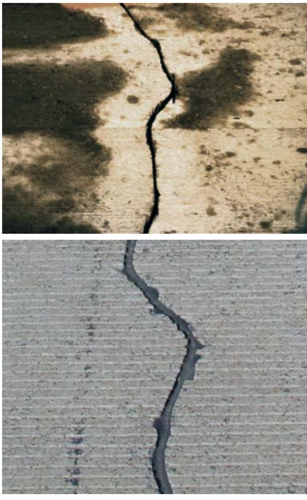
Figure 10-5. Application of joint sealant
