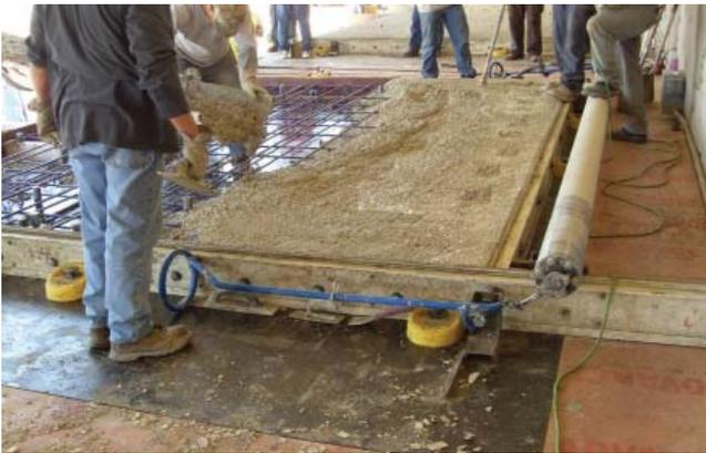
Figure 4-4. Concrete poured into form for precast panel
