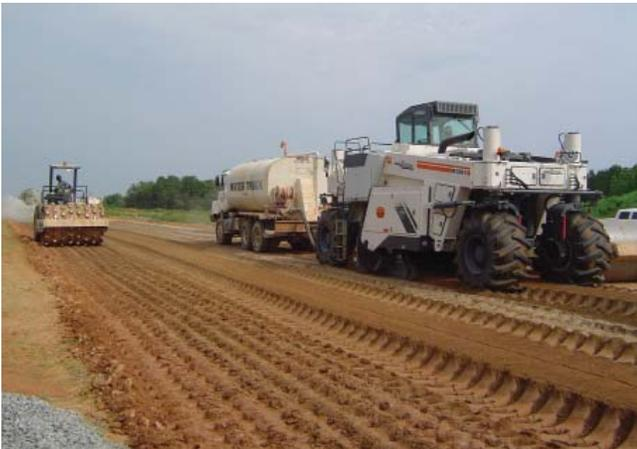
Figure 6-6. Constructing CTB using mixed-in-place method
