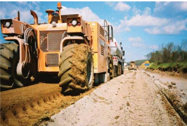
**Figure 8-3.** Pulvermizer used for in-place mixing of CMS
