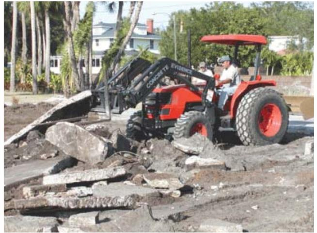
Figure 9-3. Broken concrete pavement is removed for recycling
