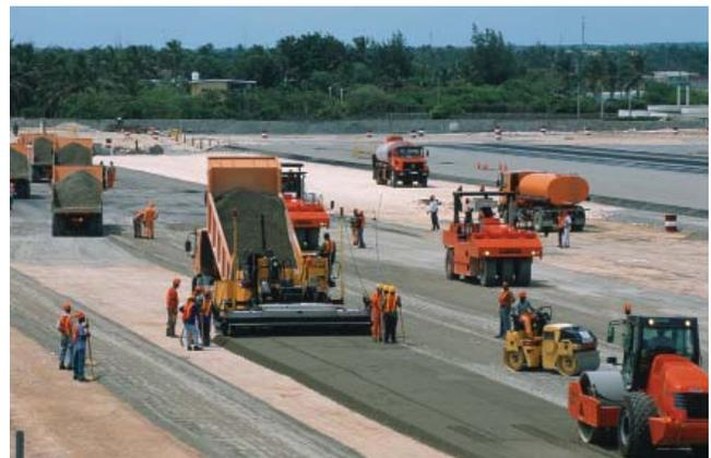
Figure 6-7. Placement of plant-mixed CTB on prepared subgrade
