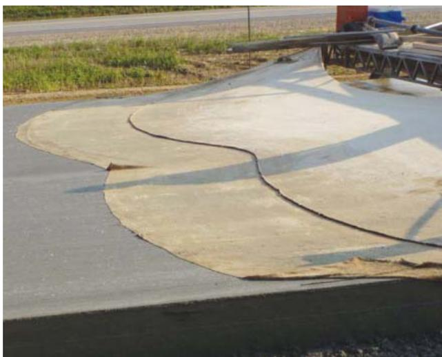
Figure 1-9. Burlap drag on fresh concrete
