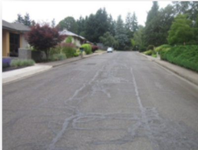
1 Street prior to construction
