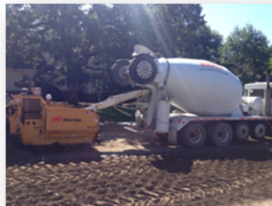
3 Discharge of cement/sand slurry
