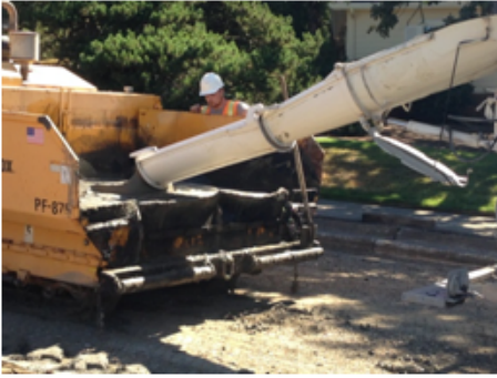
4 Discharge of cement/sand slurry
