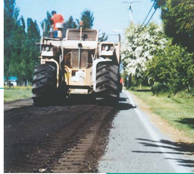
Pulverizing the old road
