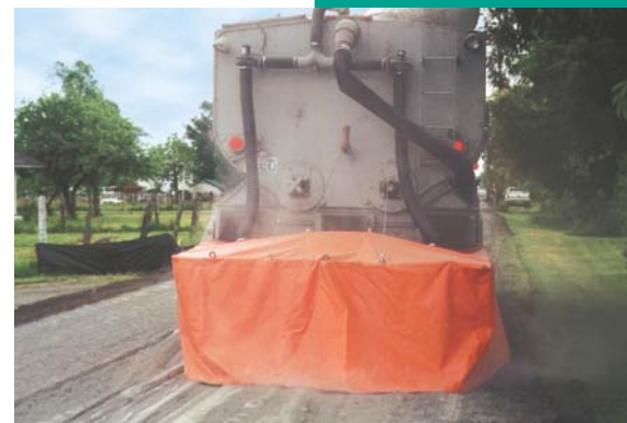
Spreading dry cement
