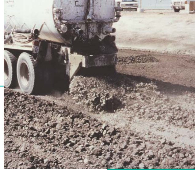
Spreading cement (slurry)
