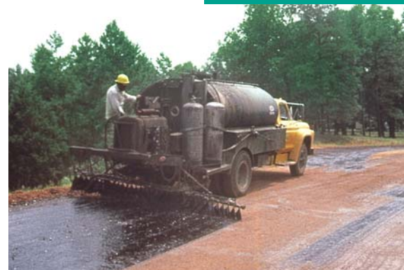
Applying tack coat prior to paving
