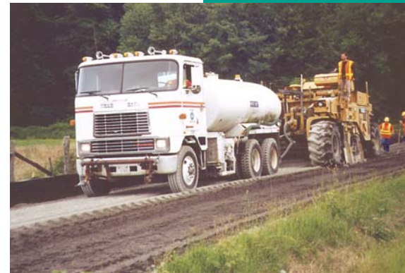
Mixing cement, soil, and water
