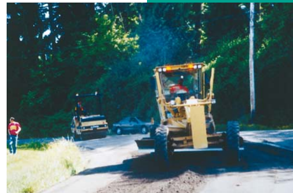
Shaping and grading
