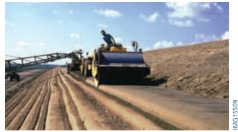
Figure 5-35. Compacting edges of soil-cement bank protection with rounded flange attached to still drum roller.
