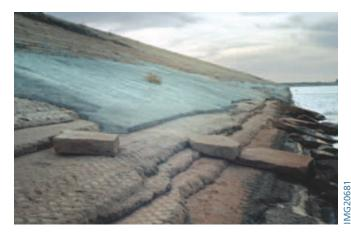
Figure 9-11. Lean concrete used to repair damaged soil-cement slope protection on Cheney Dam, Kansas.
