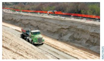
Figure 6-1. Soil-cement stream bank protection at beginning stages of construction along Santa Clara River in Valencia, California, with dewatering system in the background.
