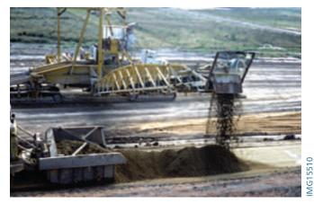
Figure 5-13. Conveyor system reduces layer width and eliminates need of earth ramps for truck travel up and down the slope.
