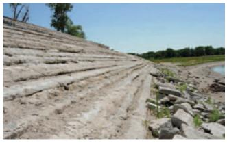
Figure 9-9. Bonny Reservoir test section in 2005 after 54 years of exposure. Drought conditions in recent years has caused the reservoir water level to drop below the toe of the soil-cement.
