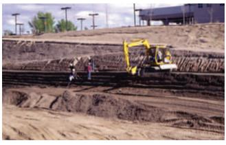
Figure 6-11. Steel plate attached to bucket of small excavator used to create and compact the vertical face of each soil-cement lift at Calabacillas Arroyo, New Mexico.
