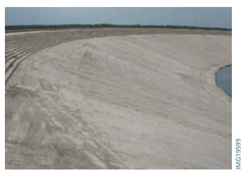
Figure 1-5. Plated and stair-stepped soil-cement slope protection at Tampa Bay Reservoir, Florida, at beginning stages of reservoir first filling.
