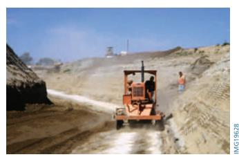
Figure 5-30. Power broom used to clean surface of soil-cement.
