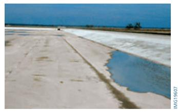
Figure 1-15. Soil-cement lined sludge lagoon in Austin, Texas.
