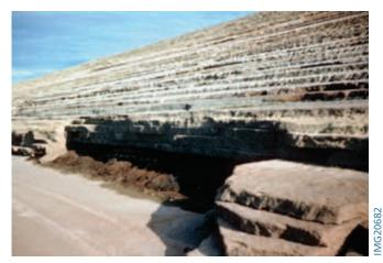
Figure 9-10. Section of soil-cement slope protection on Cheney Dam, Kansas, heavily damaged following a major storm in 1971.
