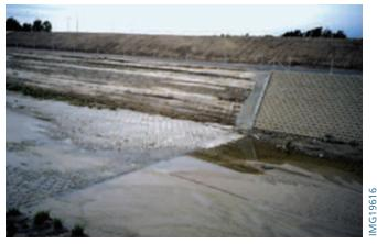
*Figure 5-9. Transition from soil-cement to concrete block bank protection, San Diego Creek, Irvine, California.*
