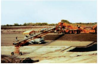
*Figure 5-15. Soil-cement placement across the slope using a paving machine.*
