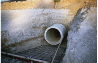
*Figure 5-7. Construction of storm drain pipe penetration in soilcement bank protection.*
