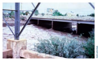
*Figure 9-4. Bridge over Santa Cruz River protected by soil-cement (shown in background) experienced no damage.*
