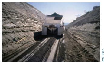
Figure 6-4. Bottom dump truck placing soil-cement, Bridgeport Project, Santa Clara River, California.
