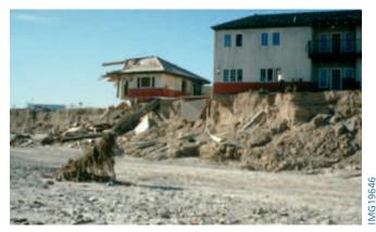
Figure 9-1. Erosion of nonprotected bank causing damage to office complex adjacent to Rillito River during 1983 flood.
