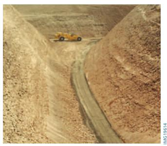
Figure 5-6. Toe excavation at upstream terminus of Tri-City Landfill soil-cement bank protection, Arizona.
