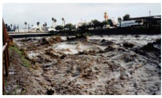
*Figure 9-3. Soil-cement shown in foreground performed well as the 1983 flood event nears its peak flow.*
