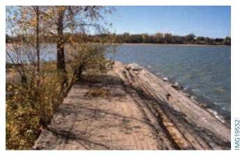
Figure 1-1. Bonny Reservoir soil-cement test section in 2001 after 50 years of service.
