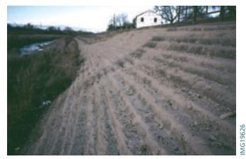
Figure 5-28. "Stair-step" edges along Sand Creek in Aurora, Colorado.
