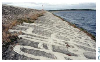
*Figure 9-14. Soil-cement bank protection (plating method) for Manatee County Dam, Bradenton, Florida, 39 years after construction.*
