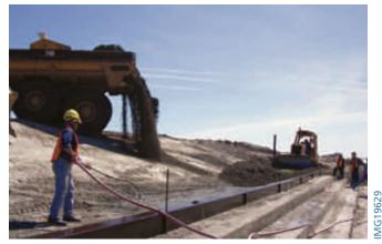
Figure 5-31. Applying cement slurry to previously placed soilcement surface immediately prior to placement of subsequent lift.
