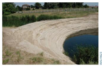
*Figure 5-24. Soil-cement grade control structure, Shop Creek, Colorado.*
