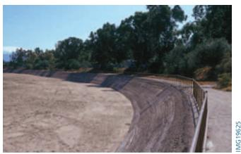
Figure 5-27. Pedestrian railing along top of soil-cement bank protection, Rillito Creek in Tucson, Arizona.
