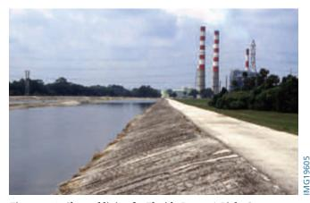
Figure 1-13. Channel lining for Florida Power & Light Company plant in Sanford, Florida.
