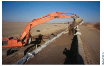
*Figure 5-12. Placement of soil-cement at Jackson Lake Dam, Colorado.*
