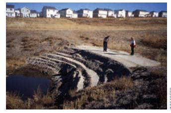
*Figure 1-17. Soil-cement drop structure constructed along Marcy Gulch, Colorado.*
