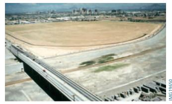
*Figure 9-8. Upstream end of CSA bank protection along Salt River at 19th Ave.*
