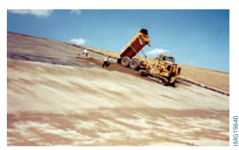
Figure 6-7. Dozer spreading soil-cement up a slope.
