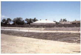
Figure 5-36. Construction of simulated geologic fault in soil-cement layers along Calabacillas Arroyo, New Mexico.
