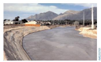
Figure 9-5. Condition of soil-cement bank protection as water recedes following 1983 flood.
