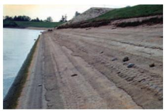
Figure 5-10. Soil-cement slope protection on Eagle Creek Dam, Indianapolis, Indiana. Note compaction marks from roller still visible 12 years after construction.
