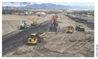
Figure 6-5. Skip bucket and excavator used to place soil-cement along Calabacillas Arroyo, New Mexico.
