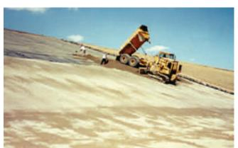
Figure 5-14. Up and down slope soil-cement placement.
