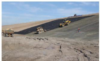
Figure 5-22. Placement of soil-cement over a geotextile fabric at Tampa Bay Reservoir, Florida.
