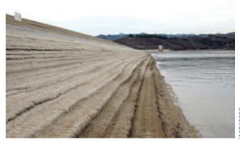
Figure 9-13. Close-up of soil-cement bank protection at Castaic Dam, California, 35 years after construction.
