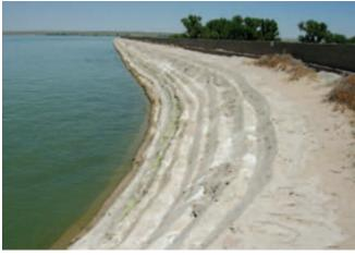
Figure 5-21. Soil-cement embankment protection with parapet wall in background, Jackson Lake, Colorado.
