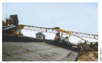
Figure 6-8. Paving machine used to spread soil-cement at Hines Energy Complex, Florida.
