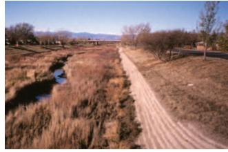
*Figure 1-10. Example of soft-bottom channel at Sand Creek, Colorado.*
