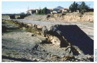
Figure 5-5. Erosion of bank material landward of soil-cement due to overtopping by flood flows, Santa Cruz River, Arizona.
