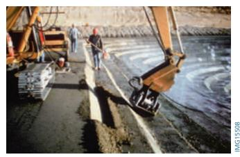
*Figure 5-34. Compacting edges with compactor attached to bucket of backhoe.*
