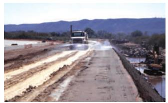
*Figure 6-12. Water truck used to prevent soil-cement surfaces from drying out.*
