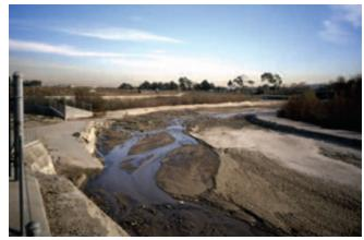
Figure 5-2. Two-tiered bank protection along San Diego Creek in Irvine, California.
