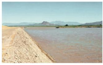
*Figure 9-6. Tri-City Landfill CSA bank protection along the Salt River.*
