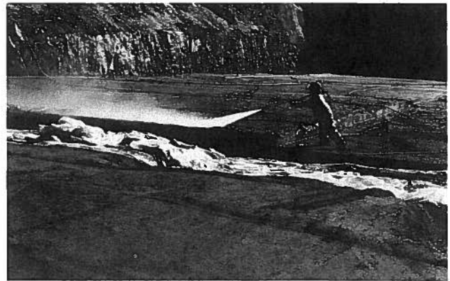
Fig. 1. Water jet blasting surface of conventional concrete foundation leveling pad prior to RCC placement at Upper Stillwater Dam, Utah.
