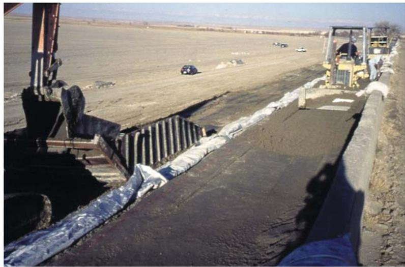
***Soil-cement placement operations adjacent to existing concrete parapet at crest of dam.***
