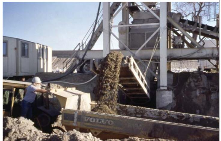
*Soil-cement batch plant located within drained reservoir.*
