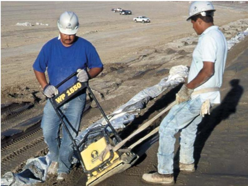
*Compacting sloping soil-cement step face with vibratory plate compactor.*
