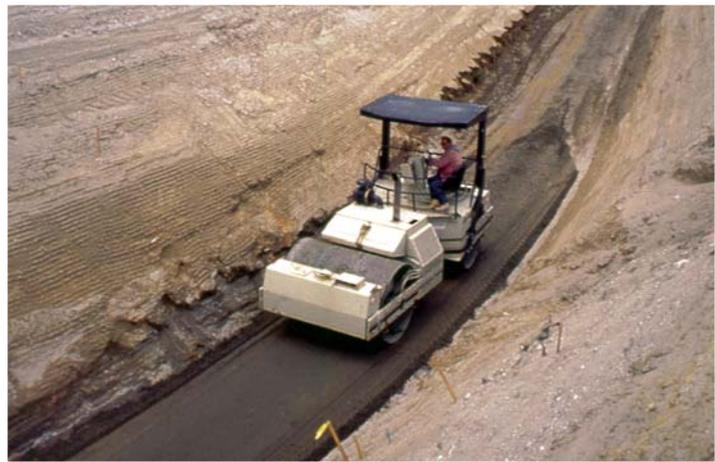
*Vibratory compactor shown compacting soil-cement lift.*
