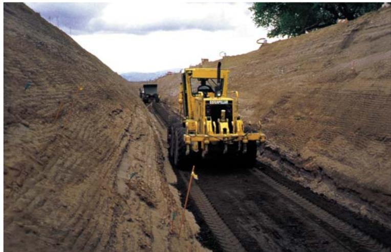
*First lift of soil-cement being spread at elevation of maximum scour depth.*
