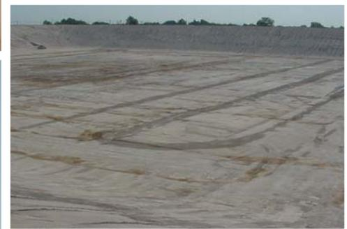
*Soil-cement shown above at normal operating pool, following reservoir refilling.*
