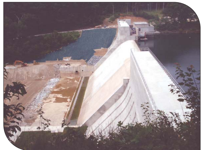
View of completed Loch Raven Dam
