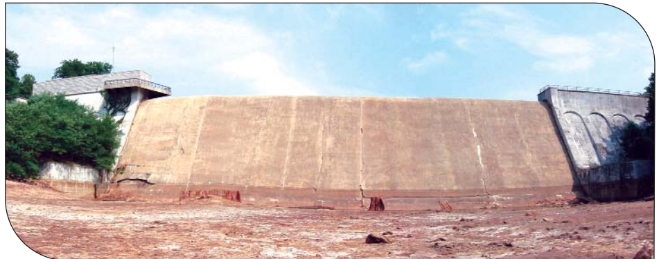
General view of Loch Raven Dam prior to rehabilitation.
