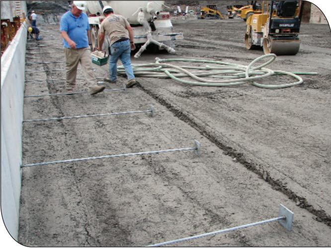
**Precast concrete upstream facing with anchoring system**
