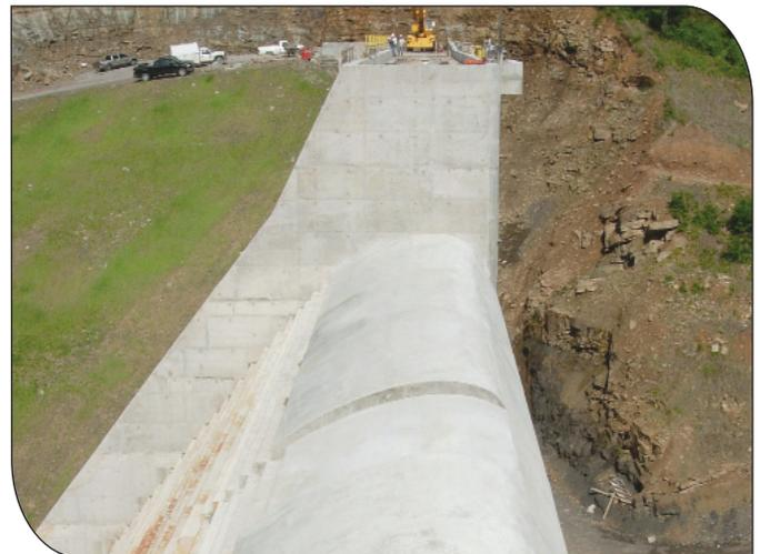
**Uncontrolled overflow spillway looking toward right abutment**
