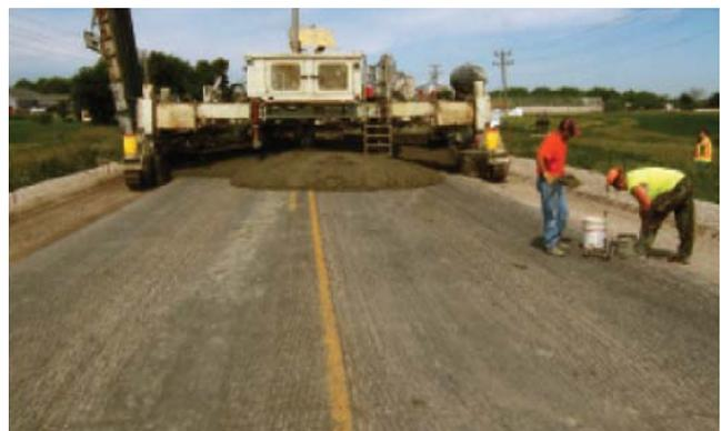
**Figure 2-5. Bonded overlay construction**
