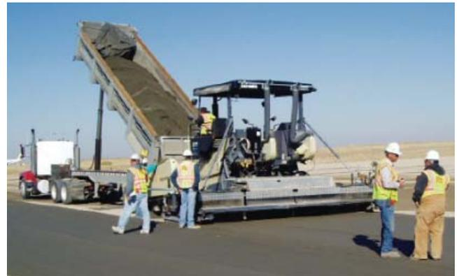
Figure 5-13. RCC placement
