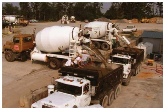
Figure 5-11 Ready-mix transit trucks dumping into haul trucks
