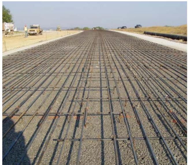
Figure 1-8. CRCP reinforcement placed before paving
