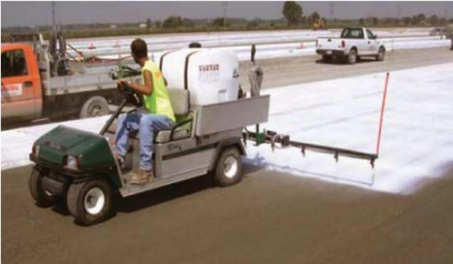
Figure 5-16. Curing RCC
