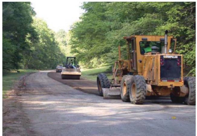
Figure 7-6. Equipment for compaction and finishing
