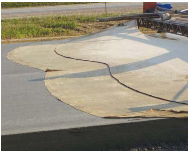
Figure 1-9. Burlap drag on fresh concrete
