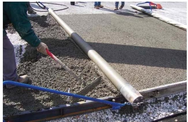
Figure 3-11. Compacting the placed pervious concrete
