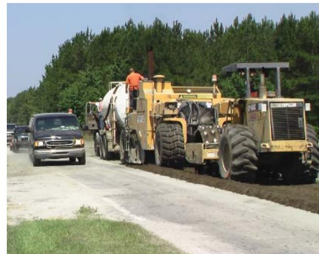
Figure 7-2 Reclaimer pulverizing existing asphalt pavement and base material
