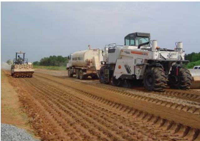
Figure 6-6. Constructing CTB using mixed-in-place method
