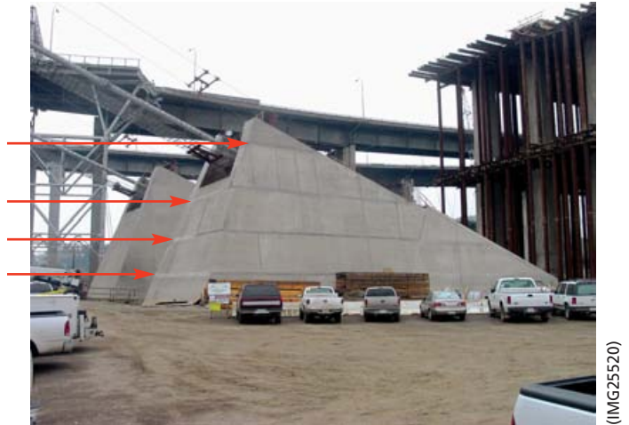
Figure 18. Bridge anchorage constructed with multiple placements (lifts are highlighted by arrows).
