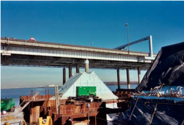
Figure 15. Insulation on bridge pier base placements; extruded polystyrene on the far pier base (left) and insulating blankets and extruded polystyrene on the near pier base (right).
