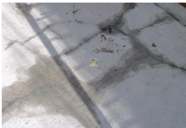
Figure 5. Thermal cracking manifested as map-cracking on the surface of a base slab.
