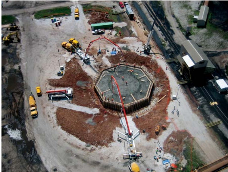
Figure 3. Placement of a chimney foundation (23.75 m [78 ft] octagon in plan, 3.1 m [10 ft] thick). (Courtesy of Chris Carson, Carson Mitchell Inc.)
