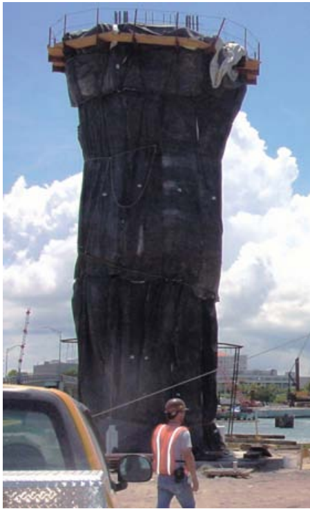
Figure 16. Concrete insulating blankets on a column.
