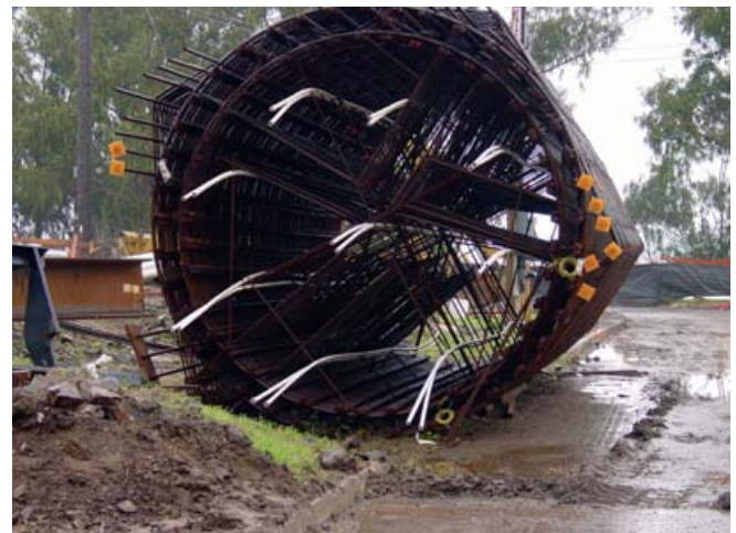
Figure 17. Cooling pipes preinstalled in a column cage.
