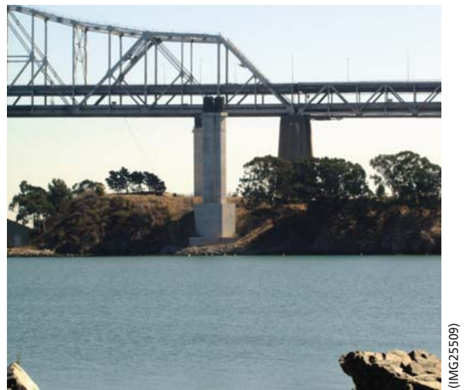
Figure 29. View of completed footing and column from across the San Francisco Bay.
