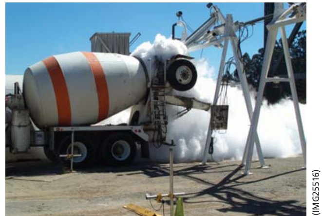
Figure 14. Liquid nitrogen precooling of concrete.
