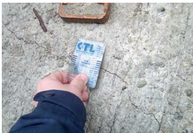
Figure 6. A more severe case of thermal cracking in a concrete footing.
