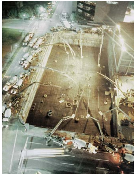
Figure 20. Planning for large mass concrete placements is essential.
