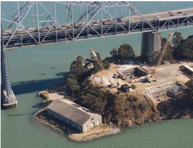
Figure 25. Partially completed excavations for the “W2.”
