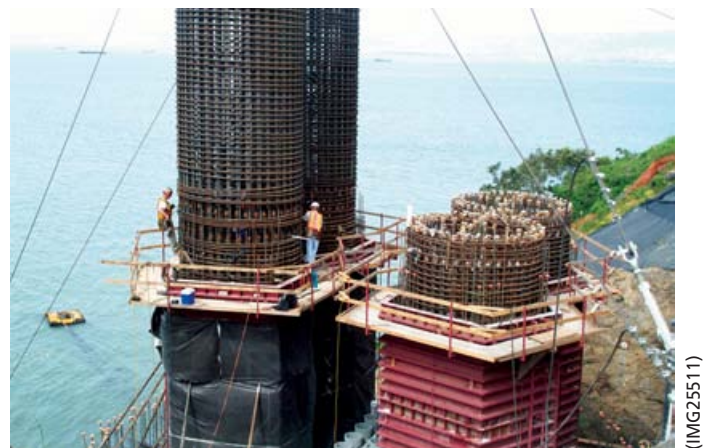
Figure 2. Mass concrete columns for the San Francisco-Oakland Bay Bridge.
