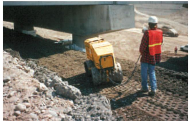
**Figure 6-10.** Remote-controlled vibratory compactor for use in inaccessible areas.
