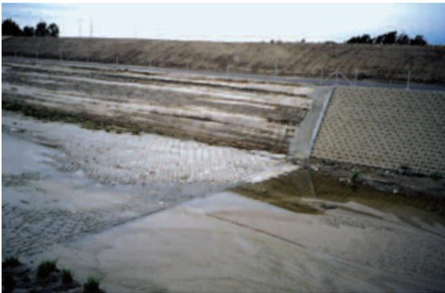
Figure 5-9. Transition from soil-cement to concrete block bank protection, San Diego Creek, Irvine, California.
