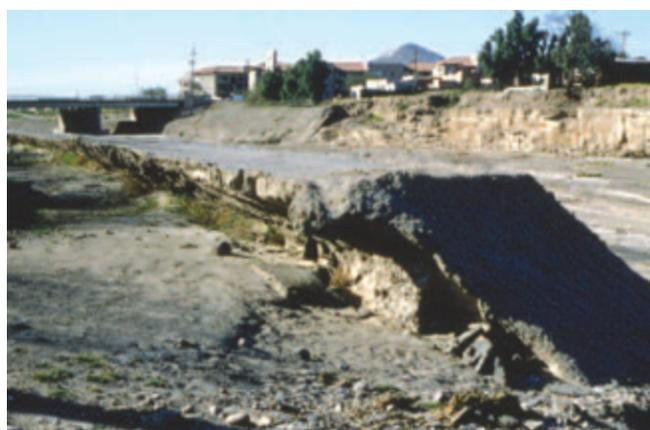
Figure 5-5. Erosion of bank material landward of soil-cement due to overtopping by flood flows, Santa Cruz River, Arizona.
