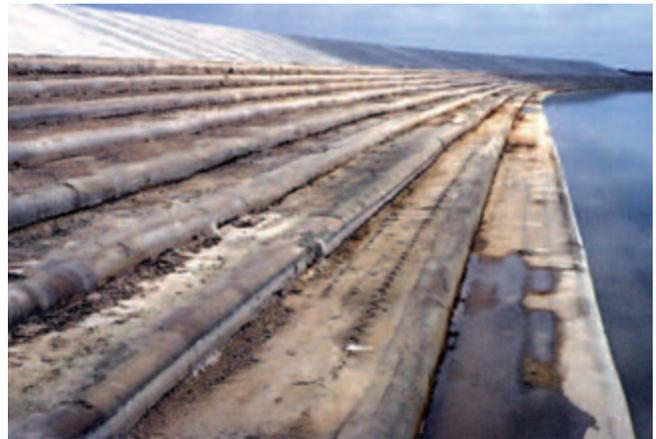
Figure 1-3. Completed “stair-step” slope protection project, Texas.
