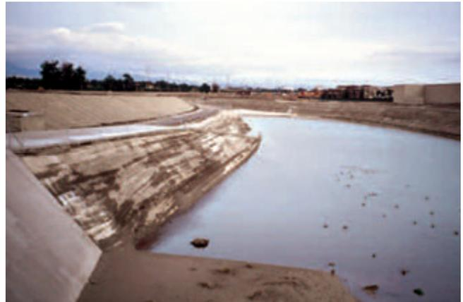
Figure 1-11. Example of trimmed smooth soil-cement bank protection along San Diego Creek in Irvine, California.
