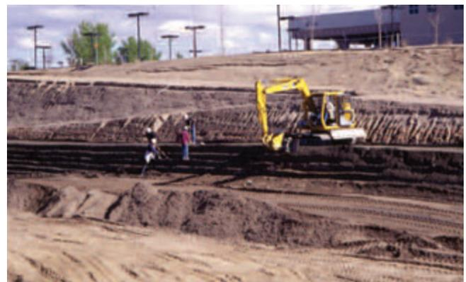
**Figure 6-11.** Steel plate attached to bucket of small excavator used to create and compact the vertical face of each soil-cement lift at Calabacillas Arroyo, New Mexico.
