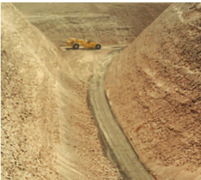
Figure 5-6. Toe excavation at upstream terminus of Tri-City Landfill soil-cement bank protection, Arizona.
