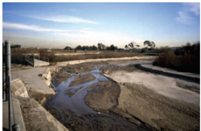
Figure 5-2. Two-tiered bank protection along San Diego Creek in Irvine, California.
