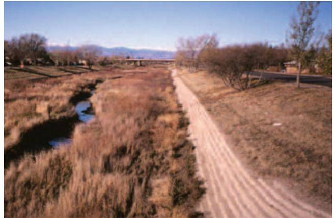
Figure 1-10. Example of soft-bottom channel at Sand Creek, Colorado.
