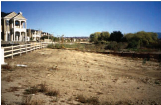
*Figure 5-38. Buried soil-cement bank protection along Santa Clara River, California.*
