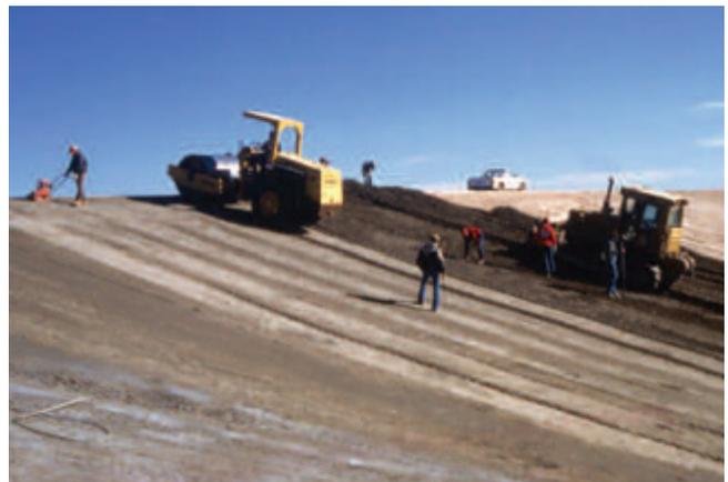
Figure 1-4. Installation of plated soil-cement slope protection.
