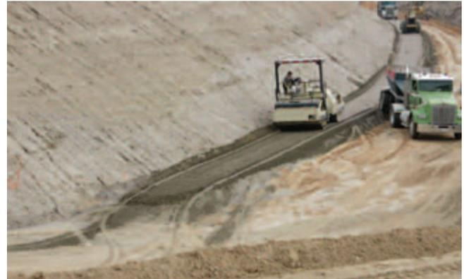
**Figure 6-9.** Vibratory roller compacting soil-cement.
