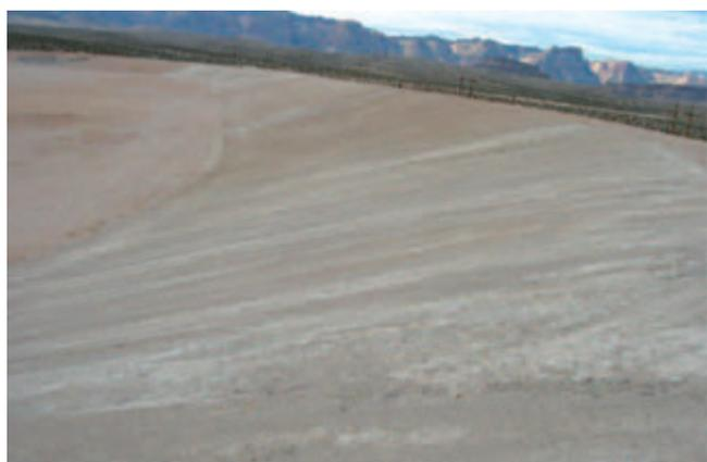
Figure 5-17. Plated soil-cement slope protection at Upper Duck Detention Basin in Clark County, Nevada.
